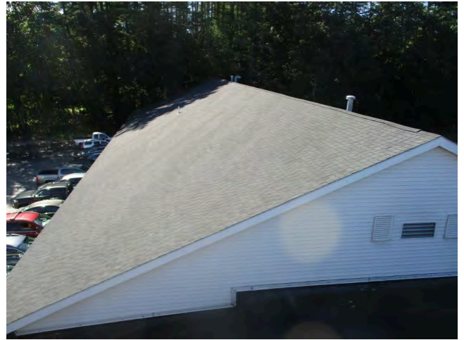
82. Roof over 2000 section view south
