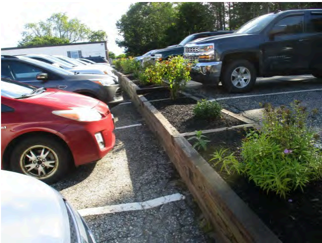
51. Retaining wall / Planters in parking area south of building
