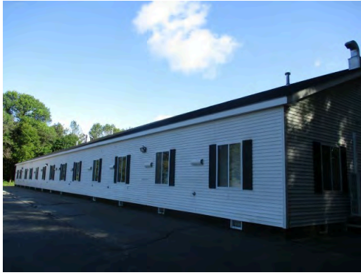
West elevation of 2000 addition
