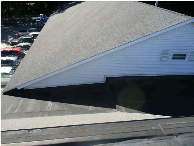
83. Roof over connector at 2000 addition
