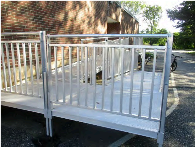
39. ADA ramp at south entrance to 1956 section
