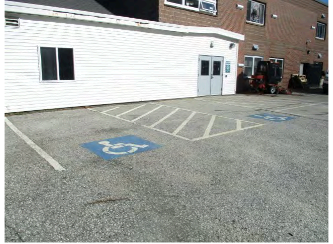
34. ADA parking south of 2000 connector corridor
