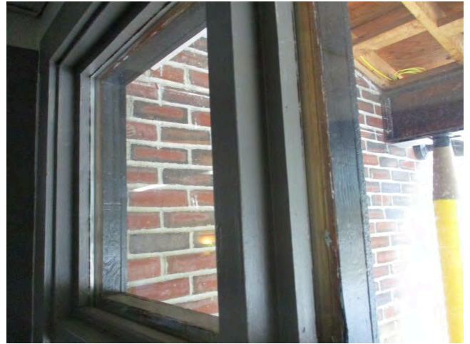
134. Windows in east end of 1956 section
