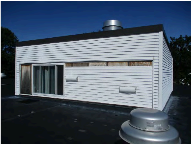
23. South elevation of office penthouse over library
