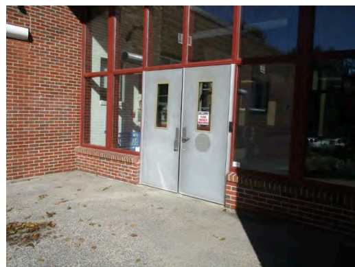
Doors at main entrance
