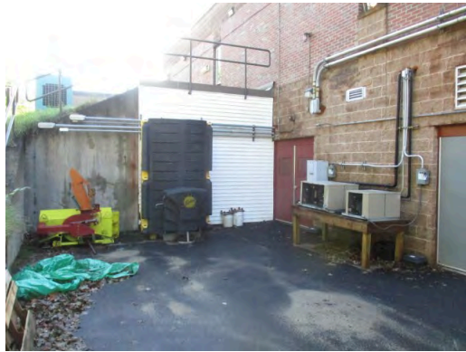
Courtyard at 1982 section boiler room and kitchen entrance showing concrete retaining wall (left)
