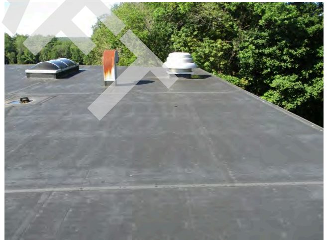
72. Roof over 1982 section view west
