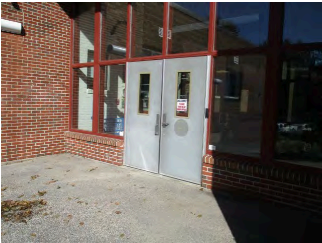
3. Doors at main entrance
