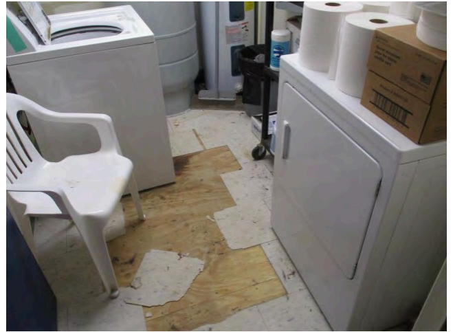
182. Utility room flooring in 2000 addition
