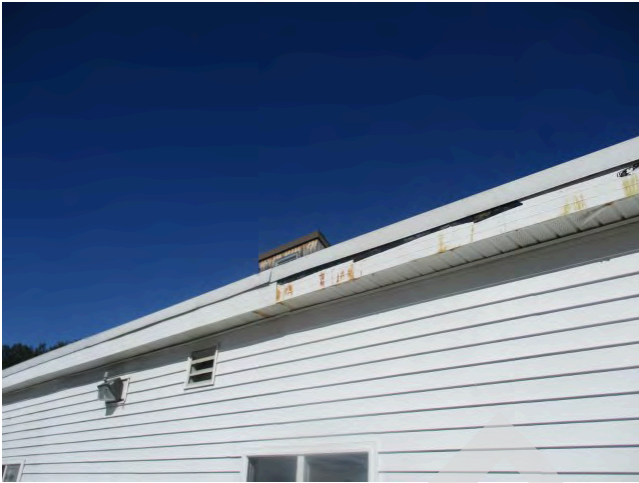
21. Soffit near entrance on south side of 2000 connector
