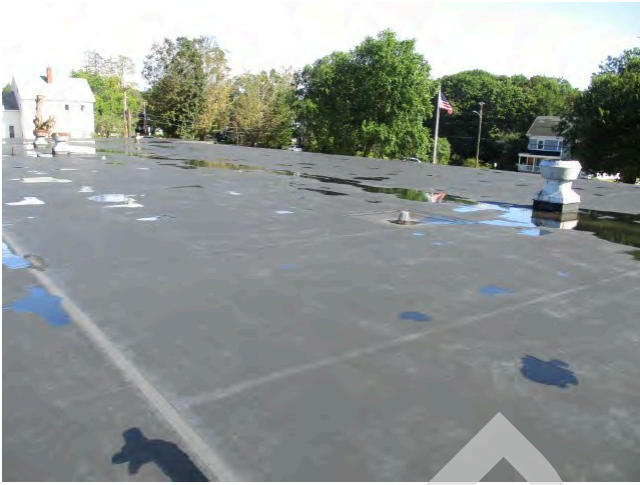
57. Roof over 1956 section view northeast
