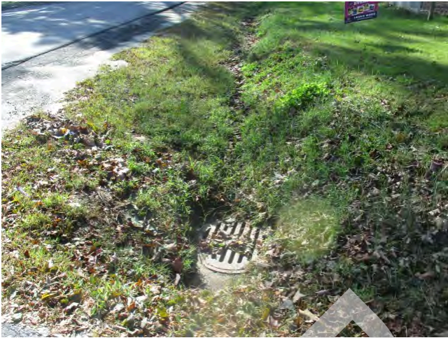
45. Catchbasin at northeast corner of Property
