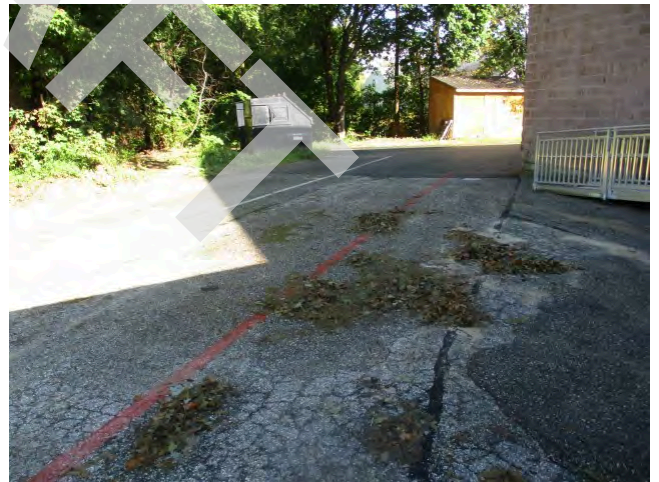
32. Pavement west of 1982 addition
