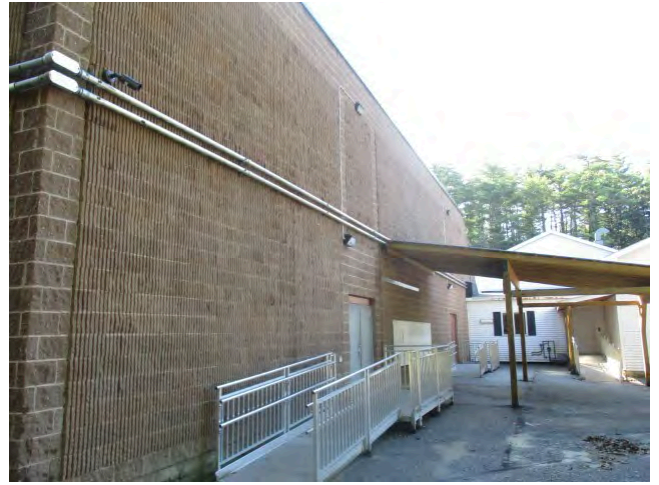
14. West elevation of 1982 section
