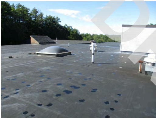
1982 roof view southwest
