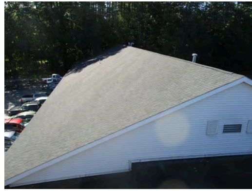
Roof over 2000 section view south
