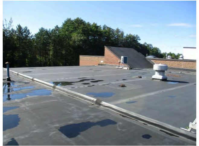
62. Roof over 1962 section view southwest
