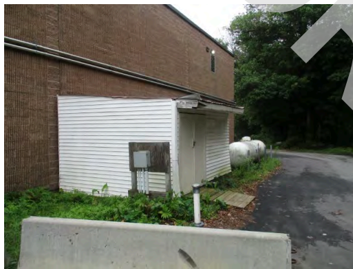
Storage shed behind kitchen
