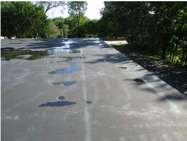
55. Roof over 1956 section view east
