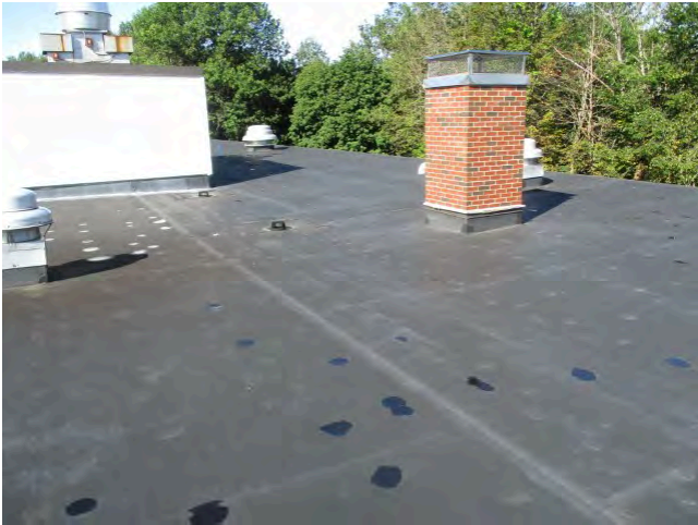
67. 1982 roof view northwest
