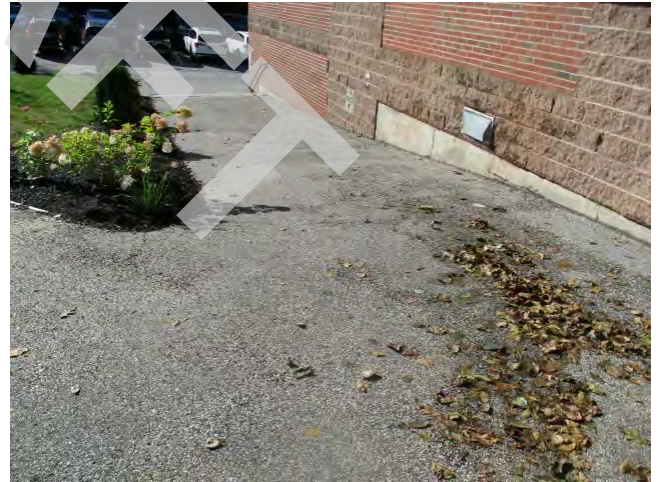
40. Walkway to main entrance
