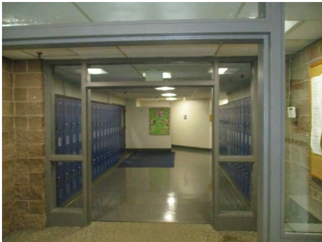
151. Corridor near gymnasium
