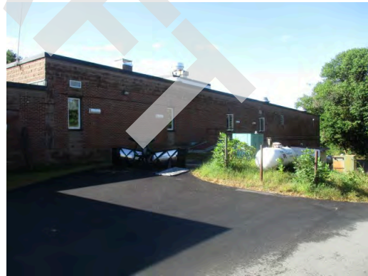
North elevation of 1982 section
