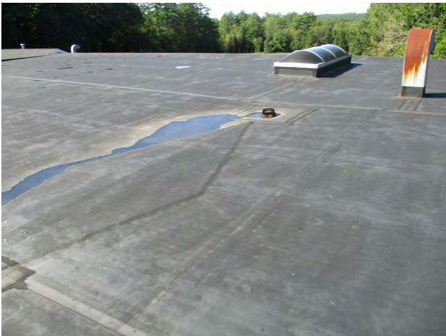
71. Roof over 1982 section view southwest
