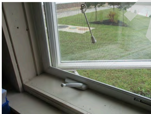
Typical window in classroom 19 in 1962 section
