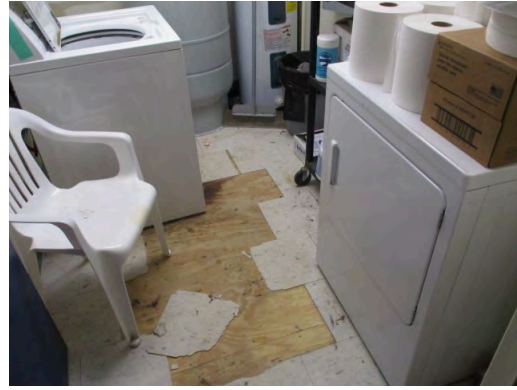
Utility room flooring in 2000 addition
