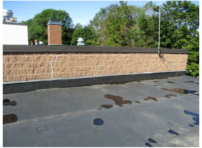
66. Kneewall at roof junction between 1962 and 1982 sections
