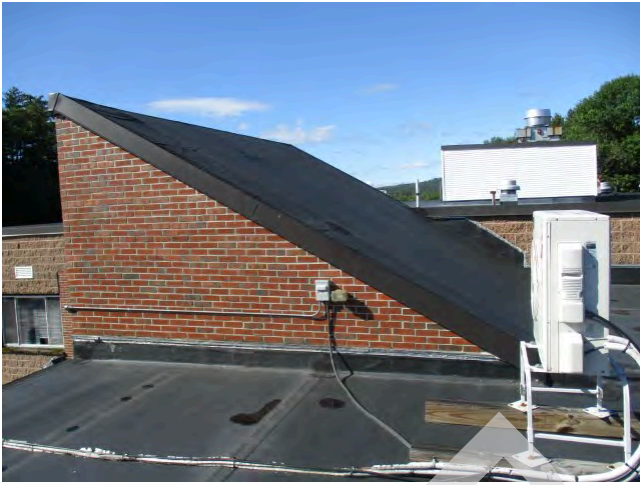
65. Roof over main entrance
