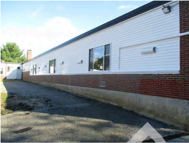
5. West elevation of 1956 section
