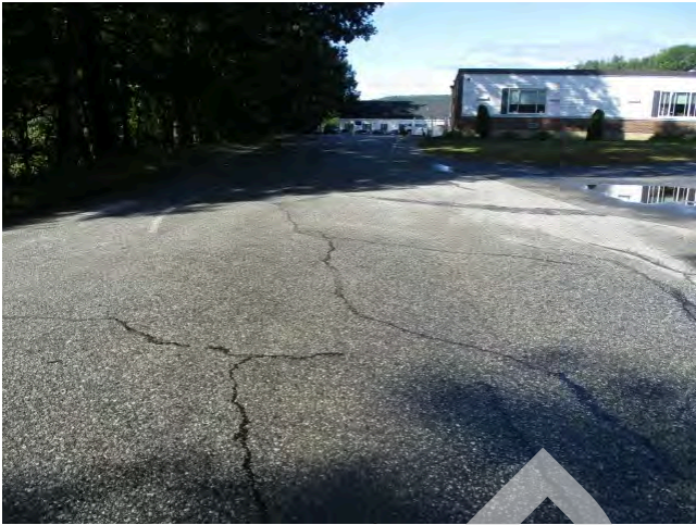
25. Pavement at south entrance from Elm Street
