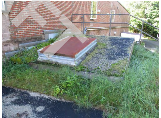
48. Bulkhead access to boiler room north of 1982 section
