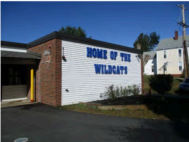
11. East elevation signage
