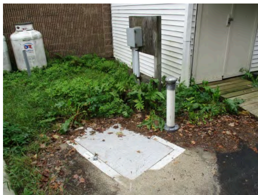
Sewer lift station behind gymnasium
