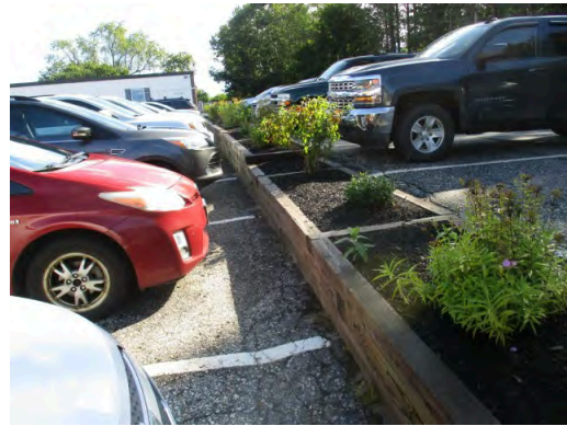
Retaining wall / Planters in parking area south of building
