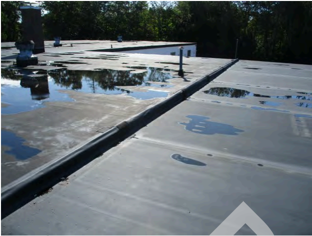
61. Roof expansion joint between 1956 and 1962 sections
