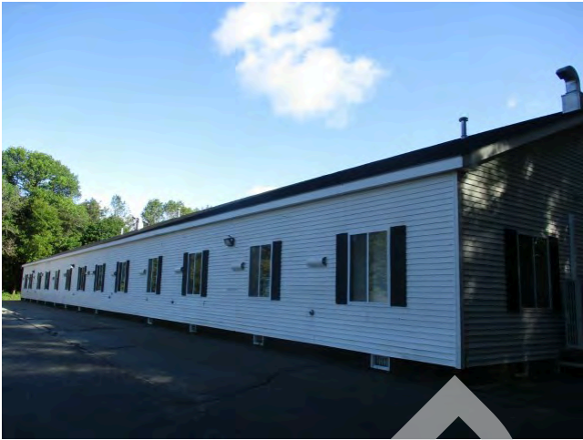
17. West elevation of 2000 addition
