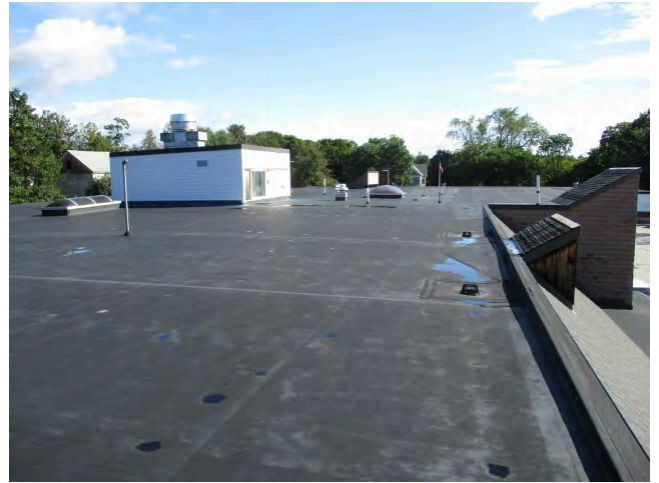
70. Roof over 1982 section view northeast
