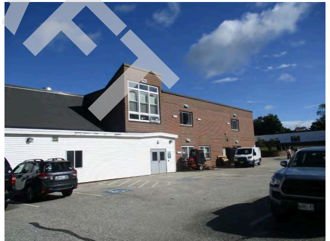
20. South elevation of 1982 addition and 2000 connector corridor
