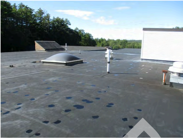
69. 1982 roof view southwest
