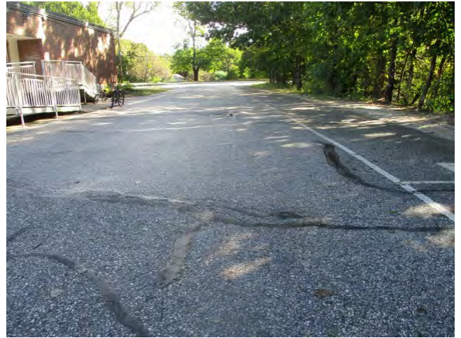
30. Pavement south of 1956 section view east west
