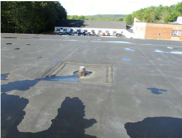
59. Roof drain over 1956 section
