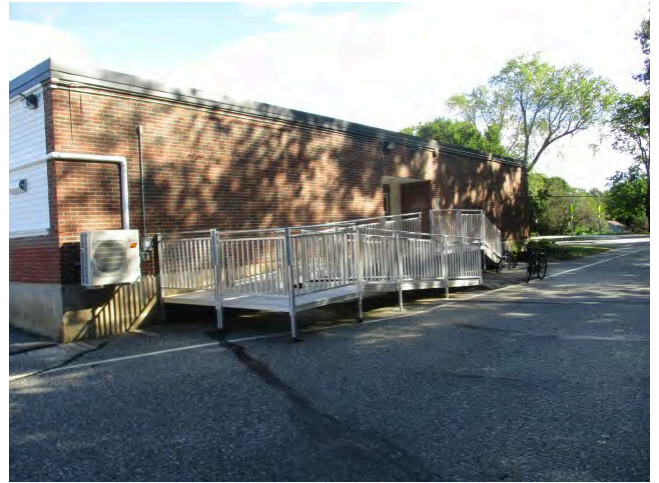
6. South elevation of 1956 section
