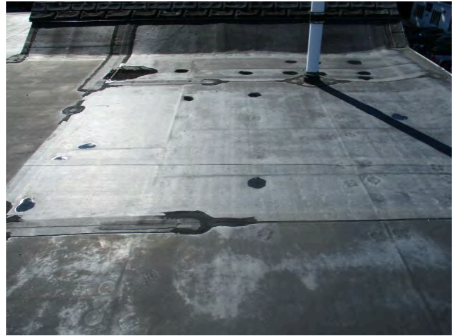
78. Replacement roof section over problem area at 1982 section and 2000 connector
