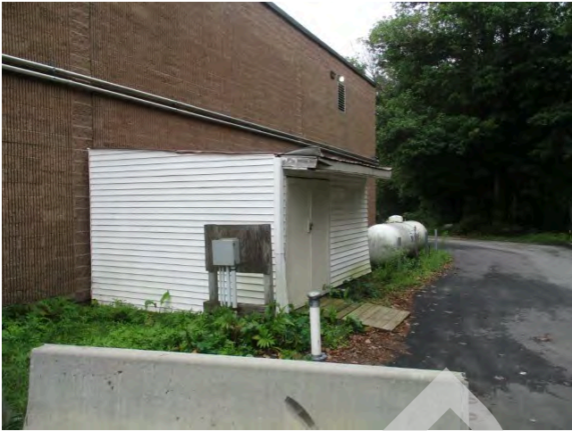
53. Storage shed behind kitchen
