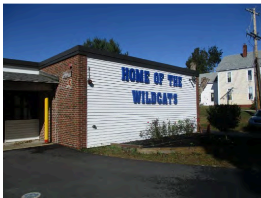
East elevation signage
