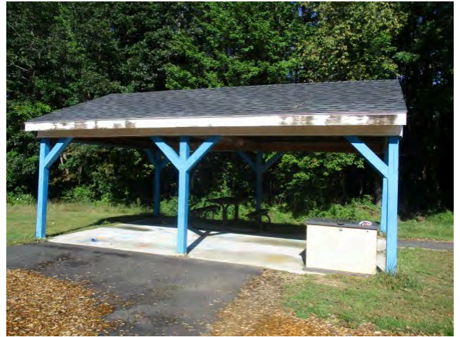
46. Outdoor pavilion west of building
