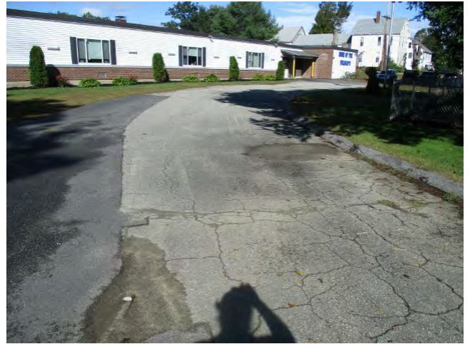
26. Pavement east of 1956 section
