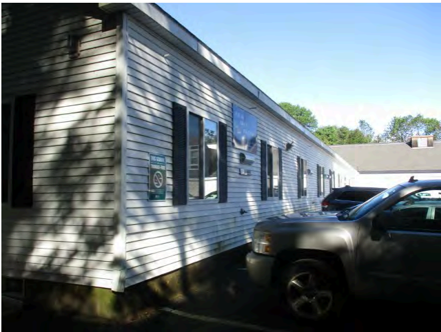
19. East elevation of 2000 addition
