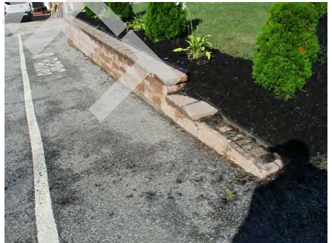
52. Retaining wall near main entrance
