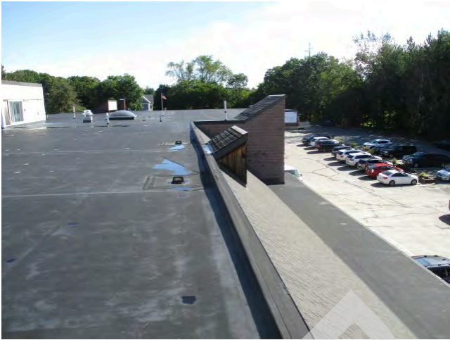
77. Roof over 1982 section, solar attic and 2000 connector
