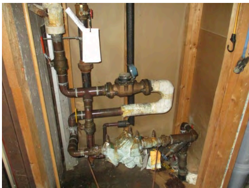
Water entrance near gymnasium
