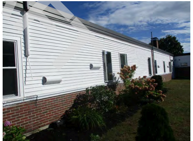
4. South elevation of 1962 & 1956 sections east of main entrance
