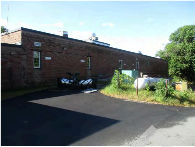
13. North elevation of 1982 section
