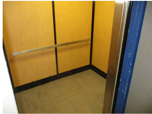
Elevator cab interior
