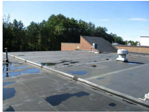
Roof over 1962 section view southwest
