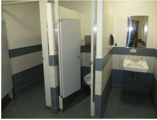
Girl's restroom near gymnasium
