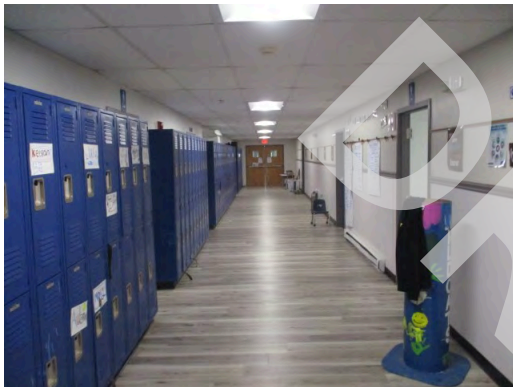
Corridor in 2000 addition
