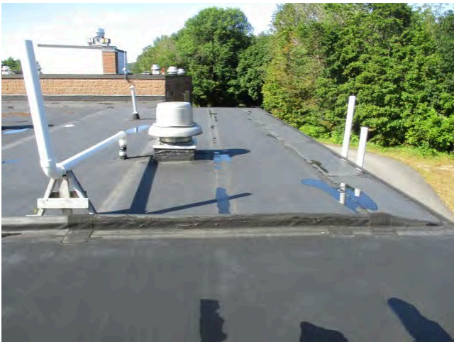
63. Roof over 1962 section view west
