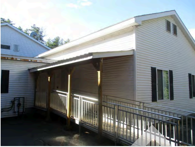
37. ADA ramp at north end of 2000 addition
