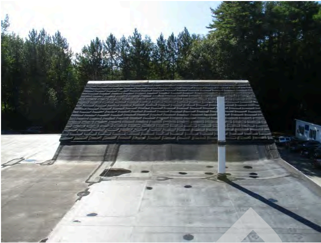
73. Roofing over classroom 28
