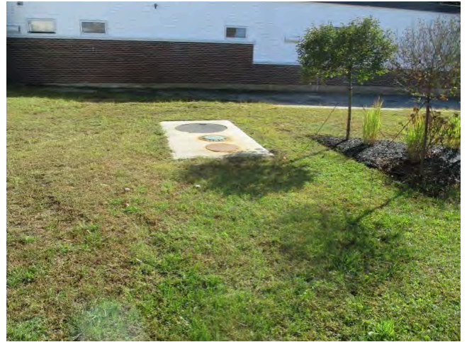
94. Heating oil UST south of 1956 section
