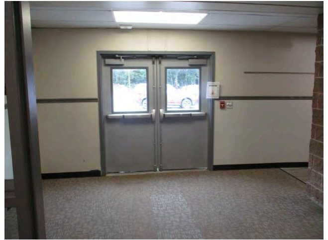
170. Doors on south side of connecting corridor to 2000 addition
