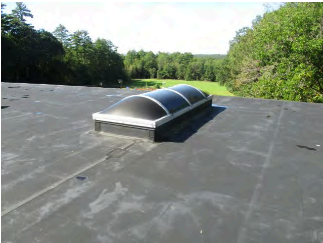
75. Skylight over gymnasium
