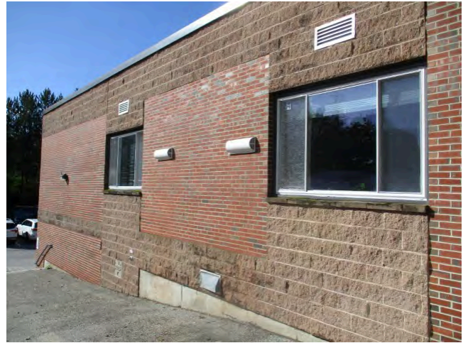
22. East elevation south of main entrance
