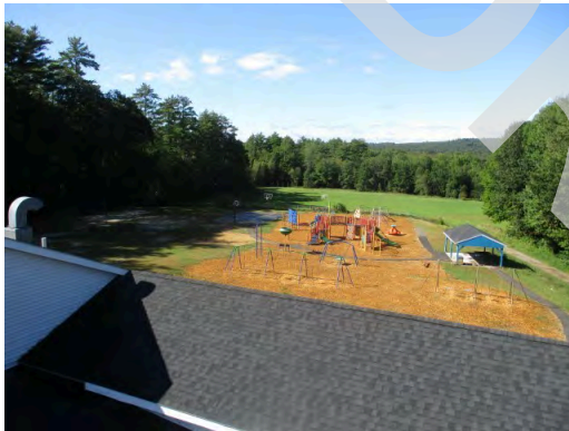
View of playground and athletic field west of building
