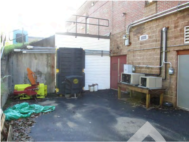
49. Courtyard at 1982 section boiler room and kitchen entrance
