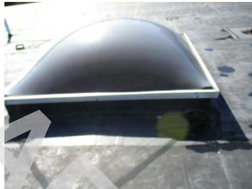
Typical skylight on 1982 roof
