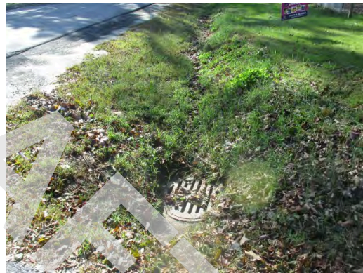
Catchbasin at northeast corner of Property
