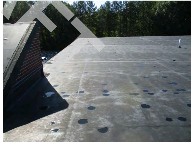
68. 1982 roof view south
