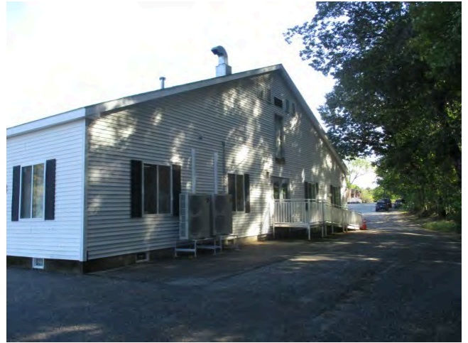
18. South elevation of 2000 addition
