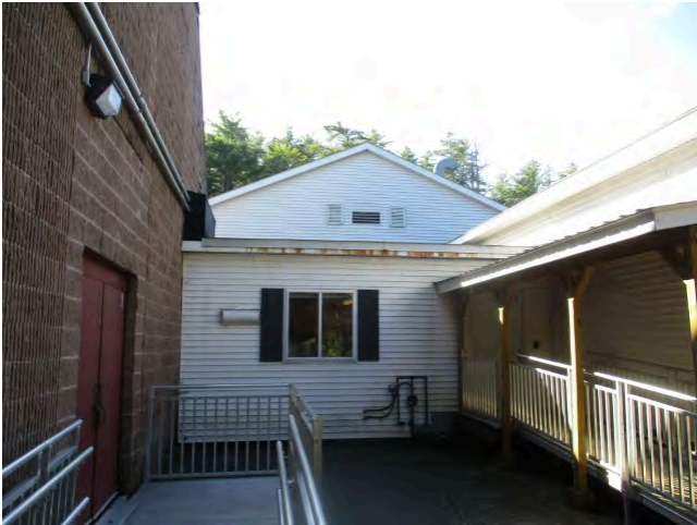
15. North elevation of 2000 connector corridor
