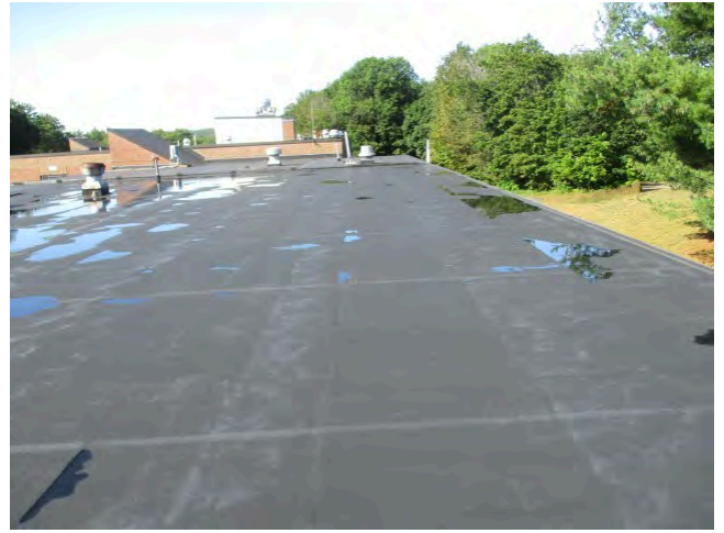
58. Roof over 1956 section view west
