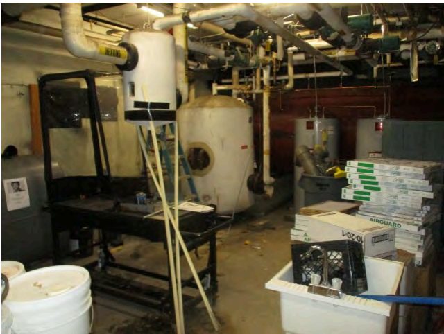
87. Boiler room near gymnasium
