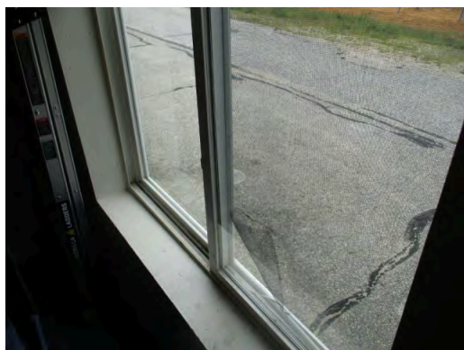
Typical window in classroom 34
