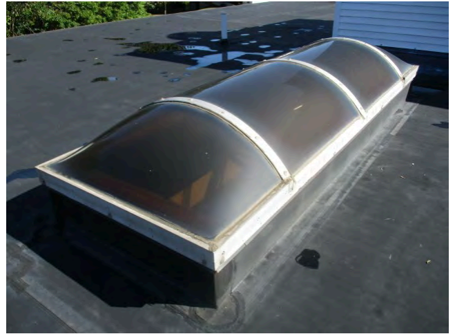
74. Roof skylight over gymnasium
