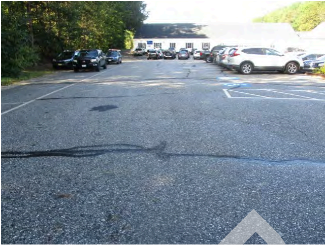
29. Pavement on south side of parking area view west
