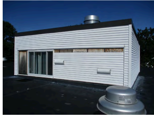
South elevation of mezzanine penthouse over library
