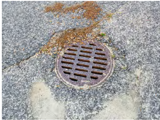
Site - Stormwater surface drains at parking areas
