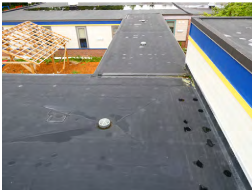
Roof - EPDM roof membrane (east facing)
