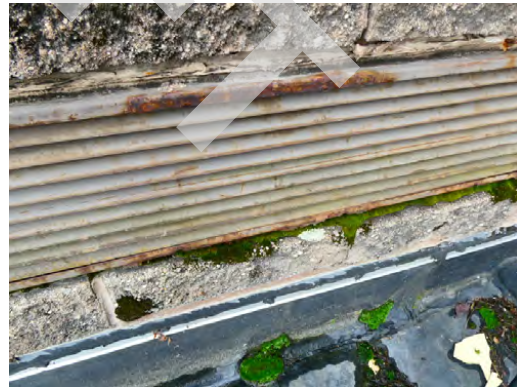
Roof - Isolated sections with organic growth present
