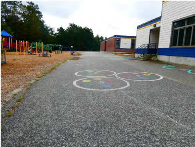
11. Site - Asphalt paved drive along north perimeter
