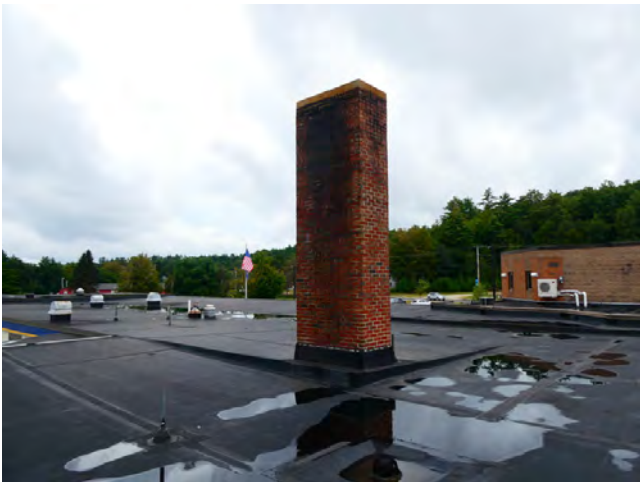
59. Roof - Brick clad chimney structure for boilers
