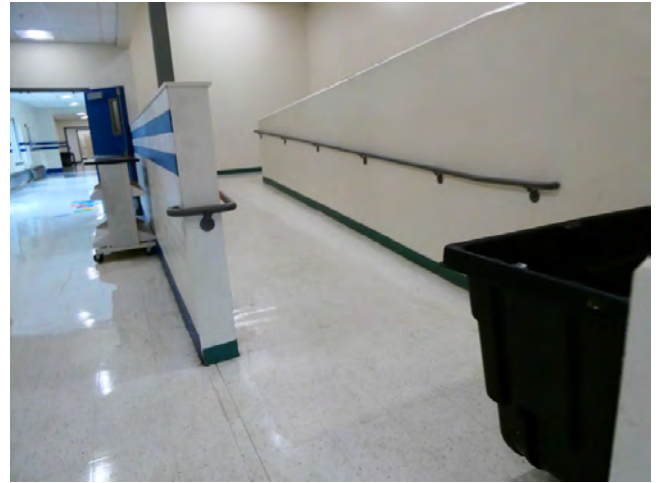
110. Interiors - Accessible ramp in northwest section
