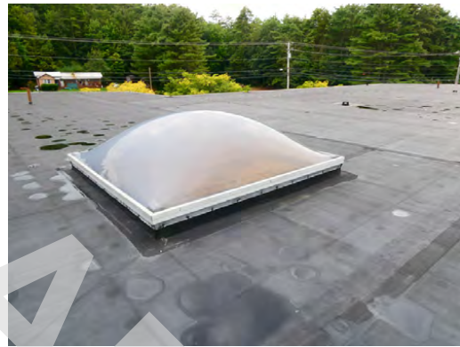
Roof - Curb mounted skylight at south roof area
