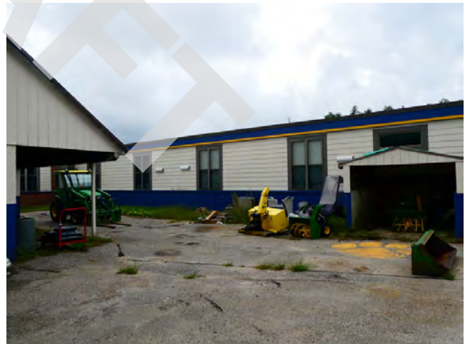
24. Elevations - North facing elevation with painted wood fiber siding
