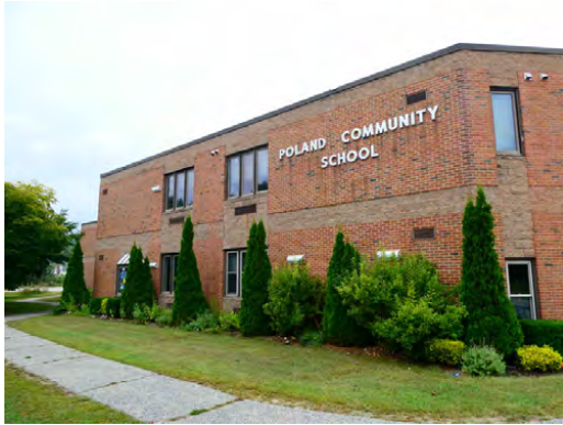
Elevations - South facing elevation and property signage
