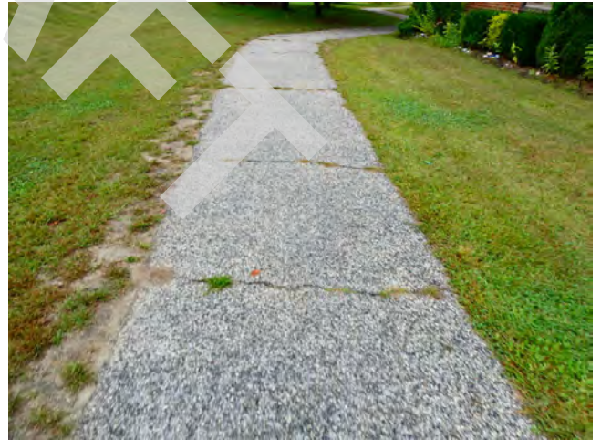
12. Site - Asphalt paved pedestrian walkways condition
