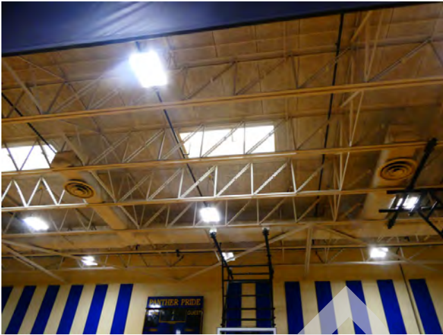
21. Structure - Open web steel joists roof framing
