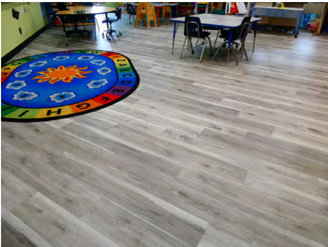
115. Interiors - New vinyl flooring in south classroom area
