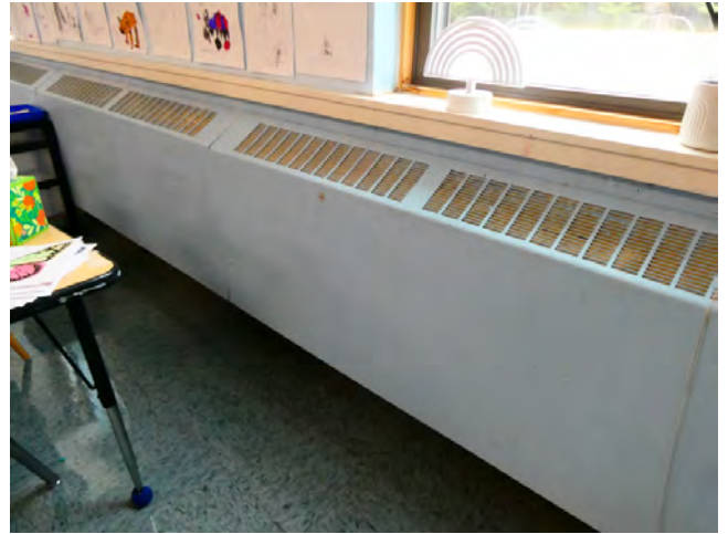
82. MEP - Wall mounted forced air cabinet unit type
