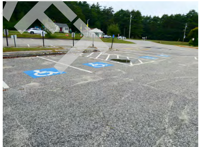
4. Site - South parking area with accessible spaces
