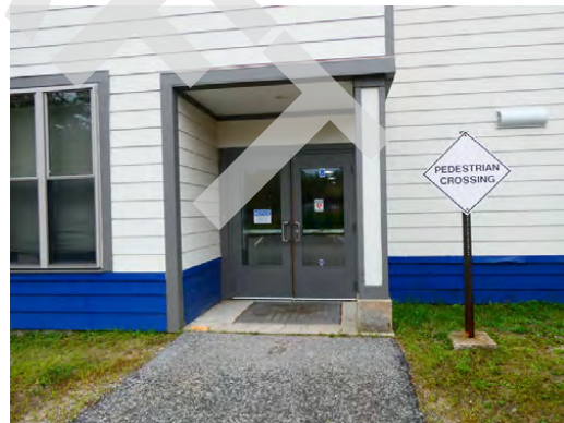
Exterior - Secondary storefront systems
