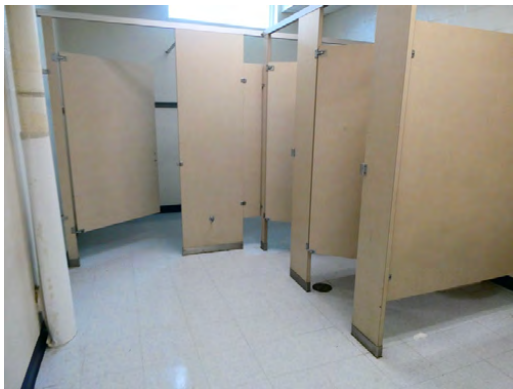
Interiors - Multi use toilet room finishes and fixtures
