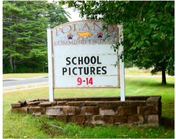
2. Site - Retaining wall with displaced/damaged sections
