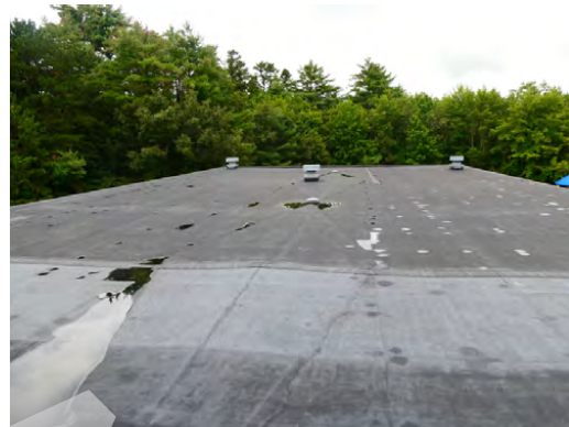
Roof - EPDM roof membrane (north facing)
