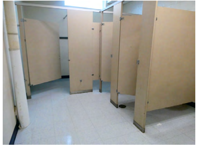
114. Interiors - Multi use toilet room finishes and fixtures
