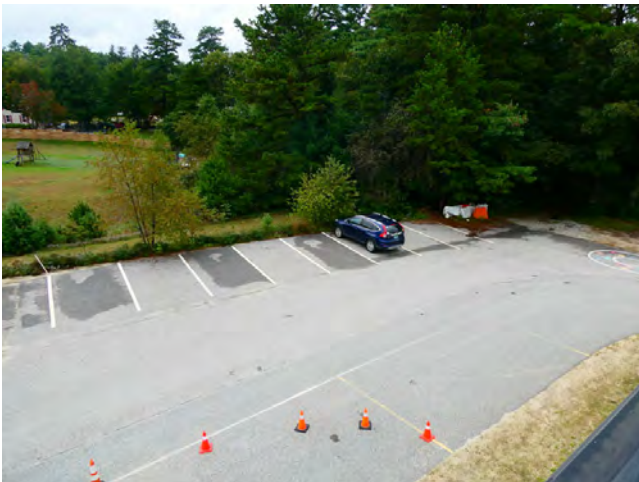
7. Site - West parking area surface
