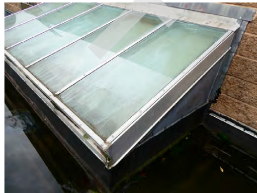
Roof - Skylight assembly at south roof area
