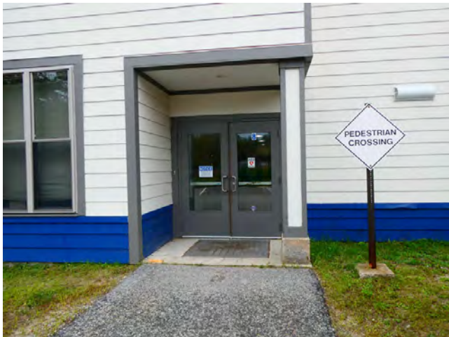
67. Exterior - Secondary storefront systems
