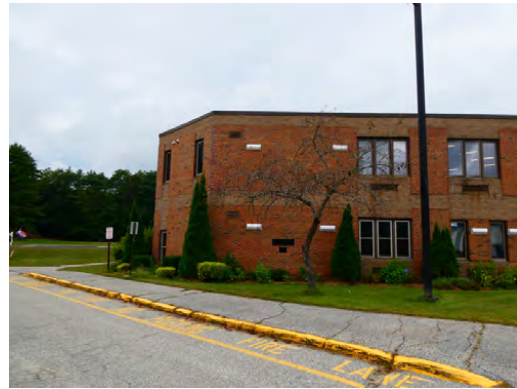
Site - Curb condition along south perimeter
