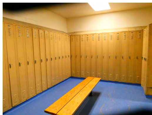
Interiors - Locker room finishes and fixtures
