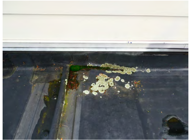
54. Roof - Isolated sections with organic growth present
