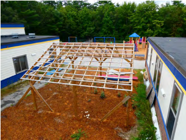
19. Site - Outdoor learning area structure under construction
