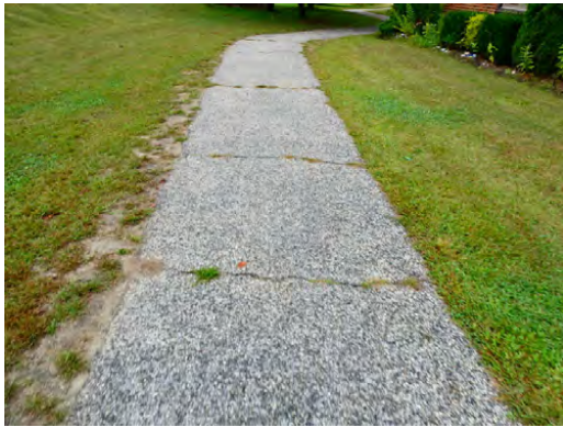
Site - Asphalt paved pedestrian walkways condition
