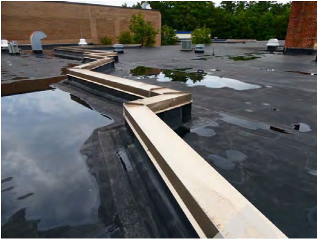
57. Roof - Parapet wall flashing type
