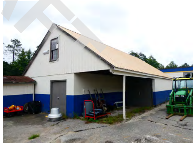
32. Exterior - Maintenance structure at north perimeter
