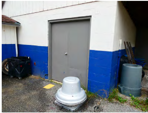
Exterior - Steel clad service door type
