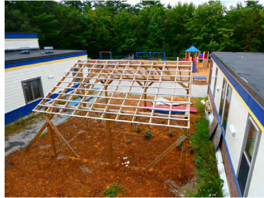
Site - Outdoor learning area structure under construction
