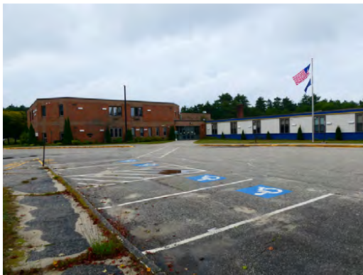
Site - South parking area condition
