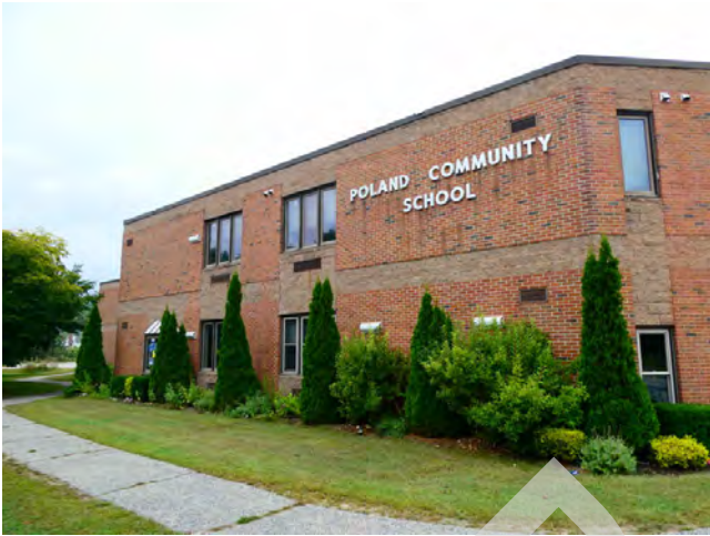
25. Elevations - South facing elevation and property signage
