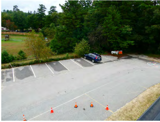
Site - West parking area surface
