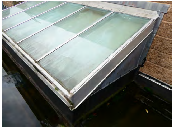
62. Roof - Skylight assembly at south roof area
