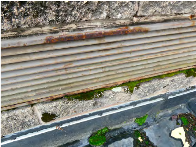
55. Roof - Isolated sections with organic growth present
