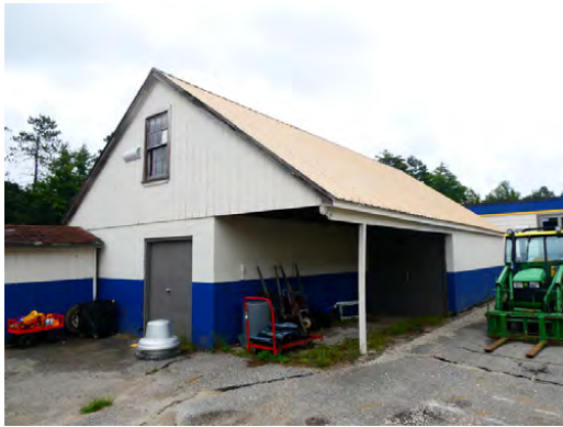
Exterior - Maintenance structure at north perimeter
