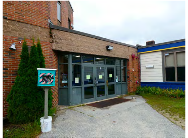
66. Exterior - Storefront system at main entrance
