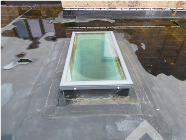
61. Roof - Newer curb mounted skylight
