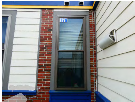
Exterior - Aluminum framed double hung windows
