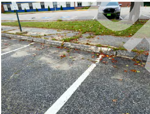
Site - Curb condition along south perimeter
