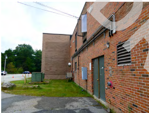
Elevations - West facing elevation and service entry
