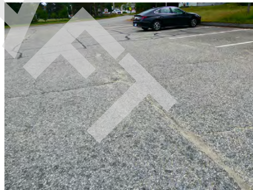
Site - South parking area condition
