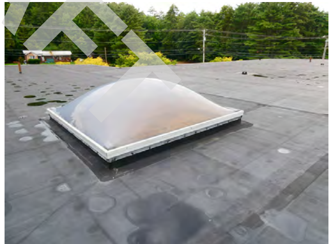
60. Roof - Curb mounted skylight at south roof area
