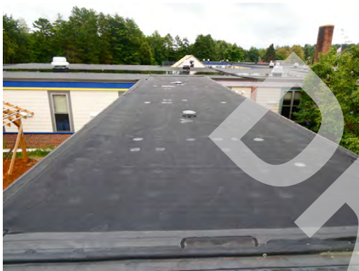
Roof - EPDM roof membrane (connecting corridor)
