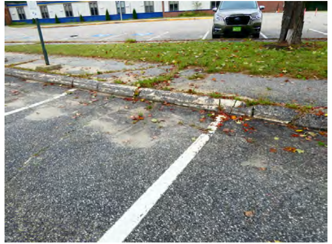
14. Site - Curb condition along south perimeter
