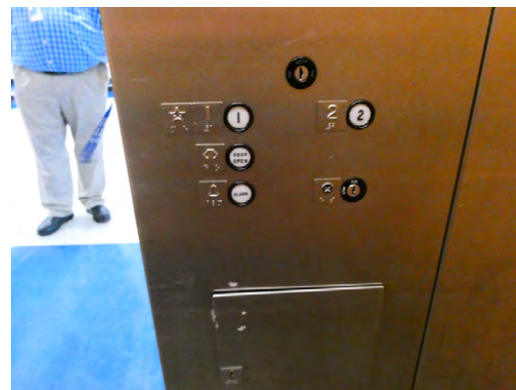
Vertical Transportation - Elevator controls
