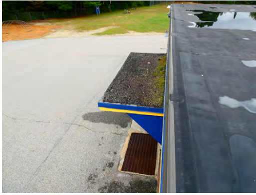
Roof - Small section of ballast covered EPDM (northeast)
