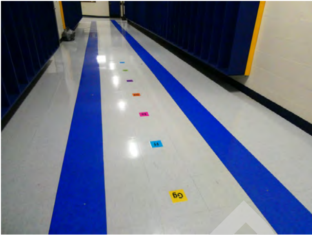
73. Interiors - Newer VCT flooring in common corridor
