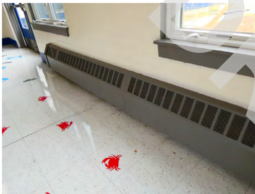
MEP - Wall mounted forced air cabinet unit type
