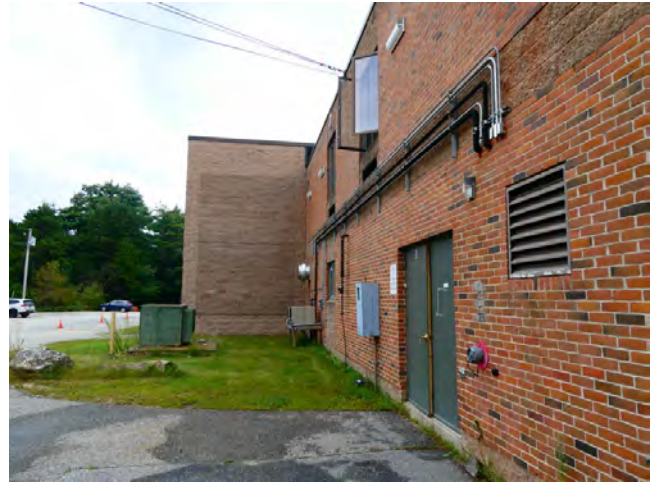
30. Elevations - West facing elevation and service entry
