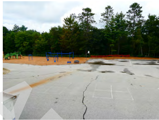
Site - North parking area and basketball court
