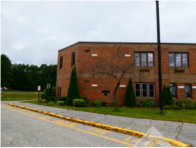
13. Site - Curb condition along south perimeter
