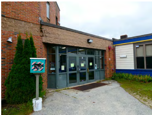
Exterior - Storefront system at main entrance
