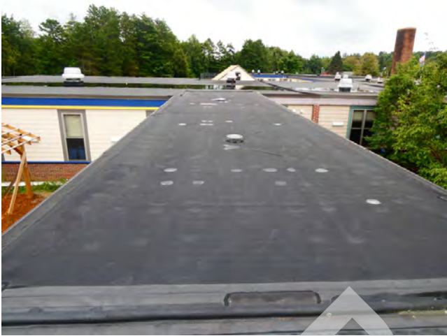
45. Roof - EPDM roof membrane (connecting corridor)
