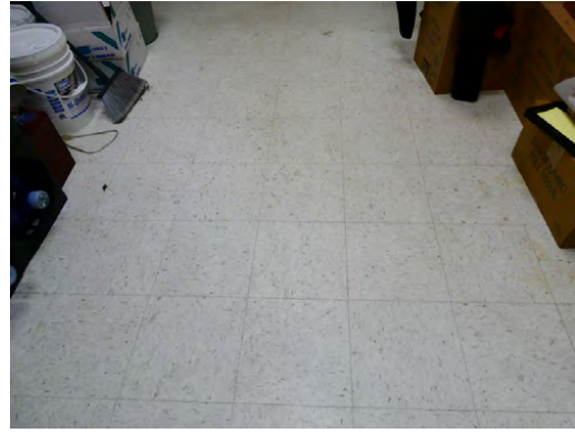
Interiors - VCT flooring type in service area
