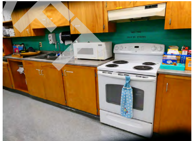
116. Interiors - Teacher breakroom area finishes and appliances
