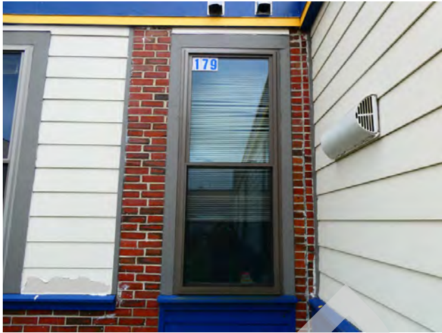
65. Exterior - Aluminum framed double hung windows
