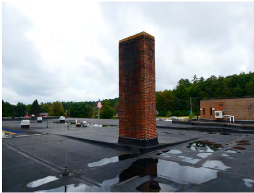
Roof - Brick clad chimney structure for boilers
