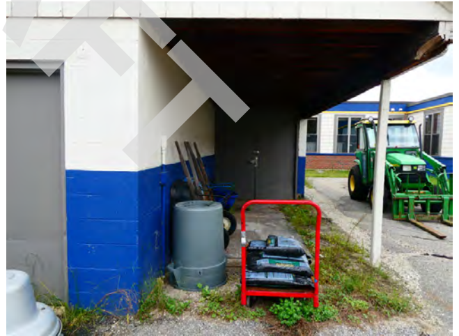
44. Exterior Painted CMU finish at maintenance structure
