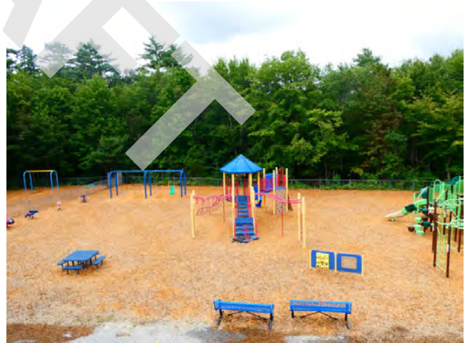
20. Site - Playground equipment along north perimeter
