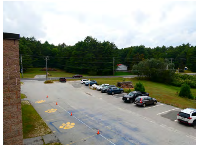
10. Site - West parking area
