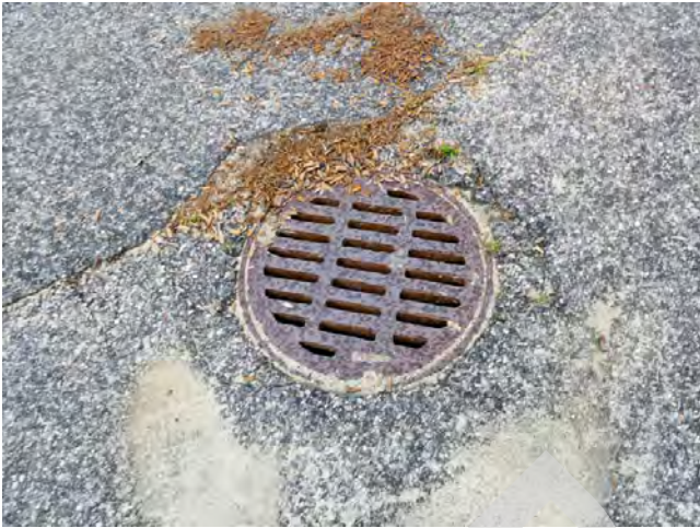
1. Site - Stormwater surface drains at parking areas
