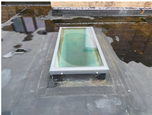
Roof - Newer curb mounted skylight
