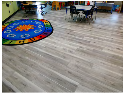
Interiors - New vinyl flooring in south classroom area
