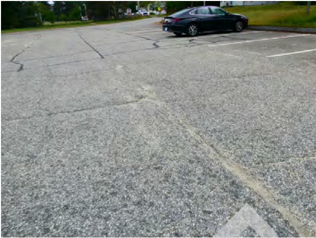
5. Site - South parking area condition
