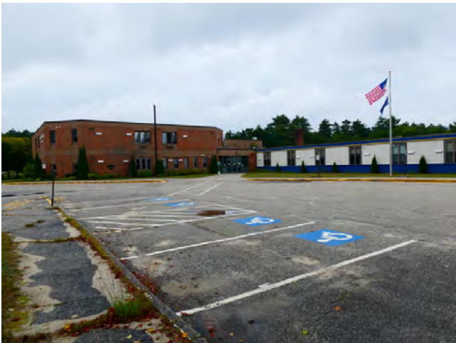
3. Site - South parking area condition
