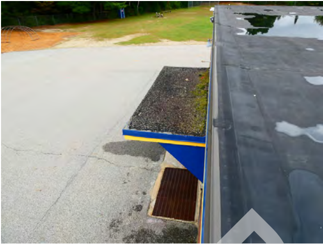
49. Roof - Small section of ballast covered EPDM (northeast)
