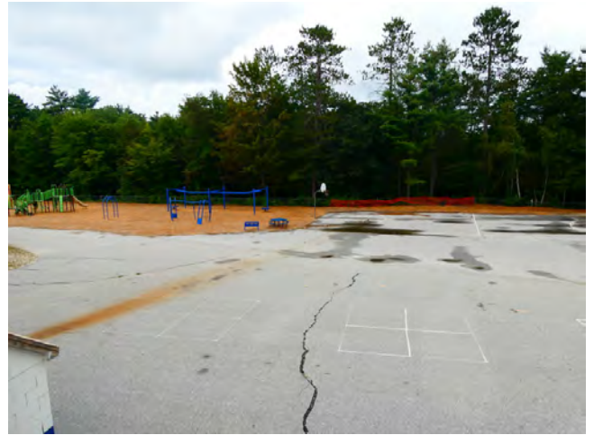
6. Site - North parking area and basketball court
