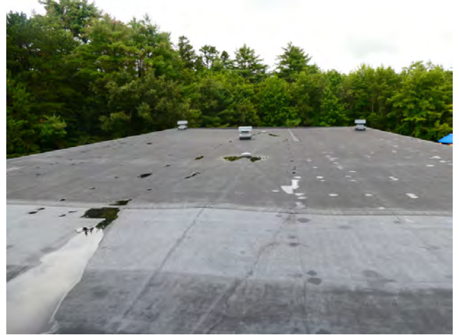
46. Roof - EPDM roof membrane (north facing)
