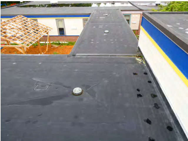
47. Roof - EPDM roof membrane (east facing)
