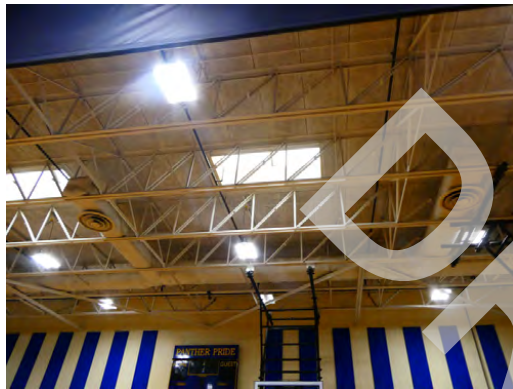
Structure - Open web steel joists roof framing
