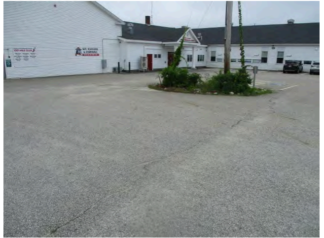
26. Pavement north of gymnasium view southwest
