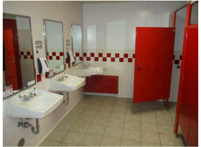
74. Boy's restroom near main office
