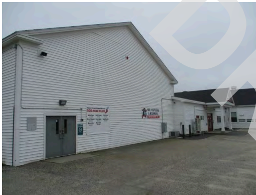
Signage at north elevation of gymnasium
