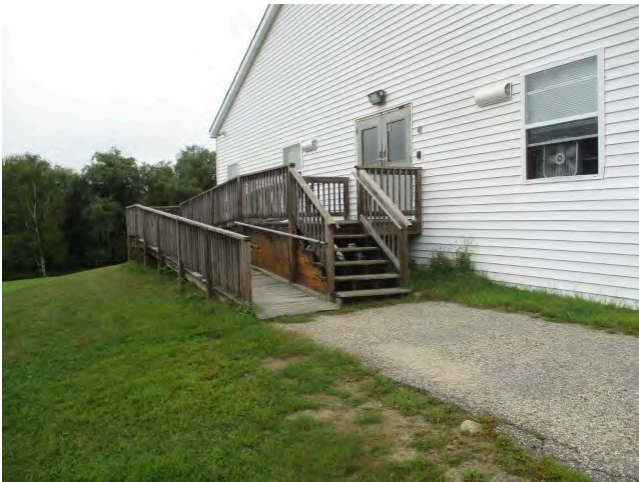
31. ADA ramp on south end of 1996 addition
