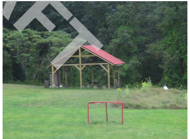
36. Outdoor pavilion on south side of Property
