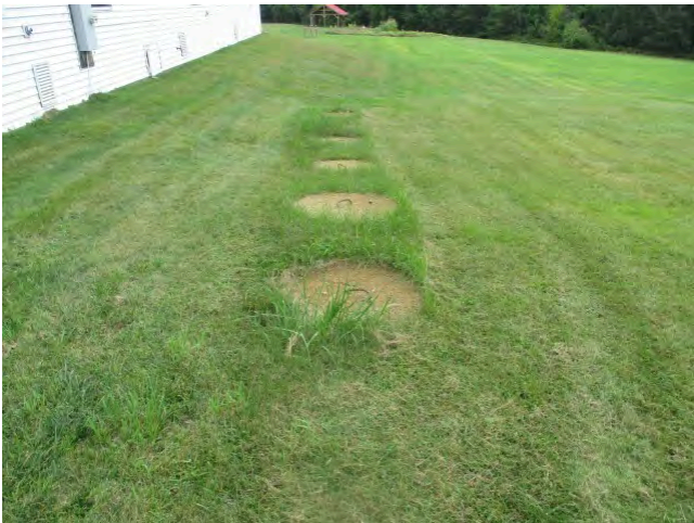
39. Septic tank west of 1996 addition
