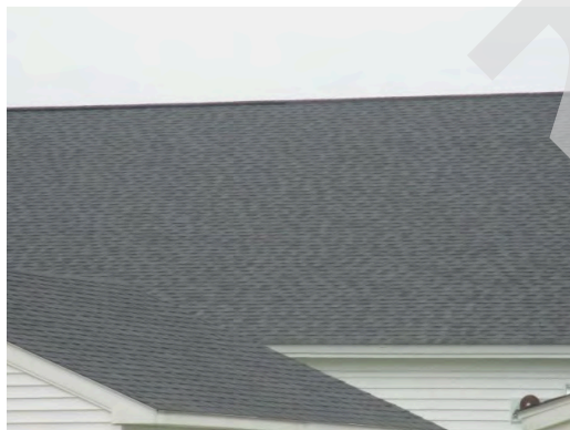
Roof over gymnasium
