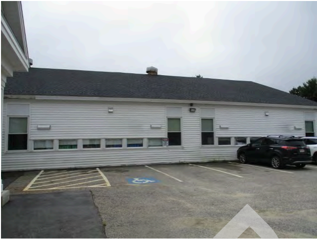
5. East elevation of north wing
