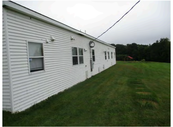
10. West elevation of 1996 addition
