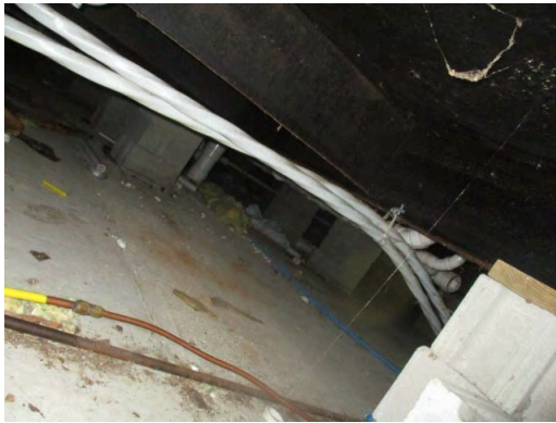
Crawlspace under 1996 addition
