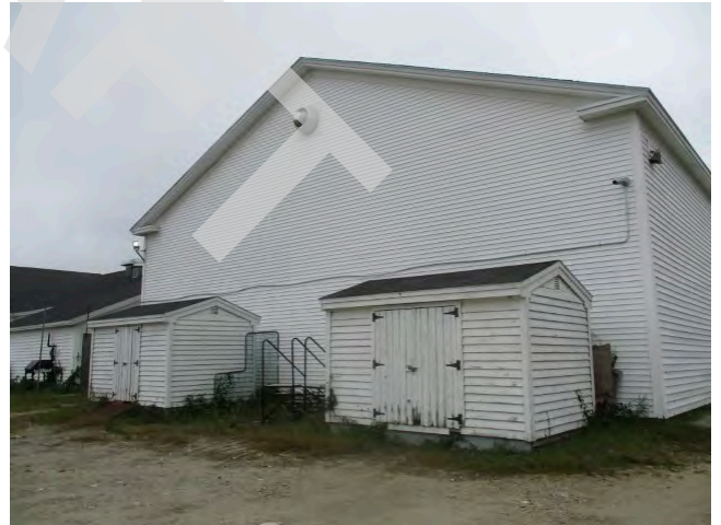
16. Storage sheds south of gymnasium
