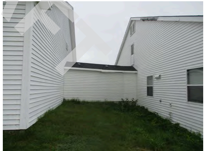
8. West elevation of connector to 1996 addition
