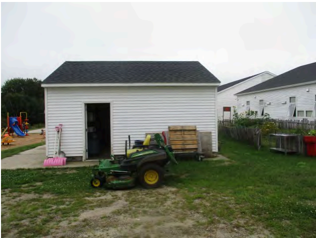
19. North elevation of maintenance building
