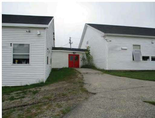
Sidewalk pavement at connector to 1996 addition
