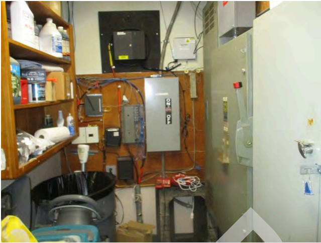
97. Janitor closet near gymnasium
