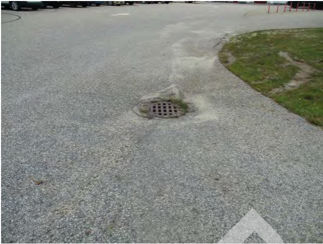
33. Catchbasin at east Property entrance
