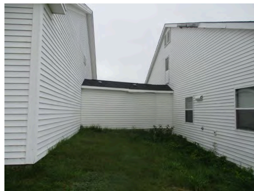
West elevation of connector to 1996 addition
