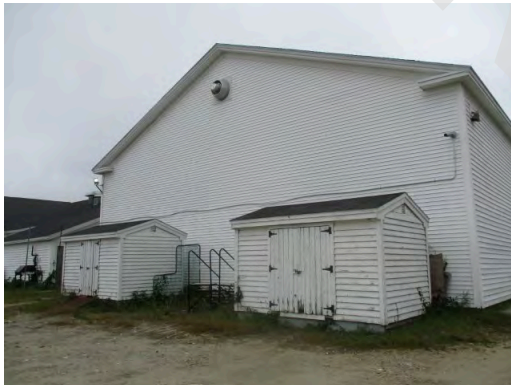
Storage sheds south of gymnasium
