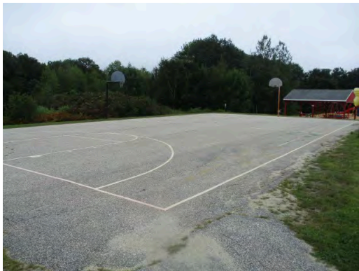
Basketball court west of 1996 addition
