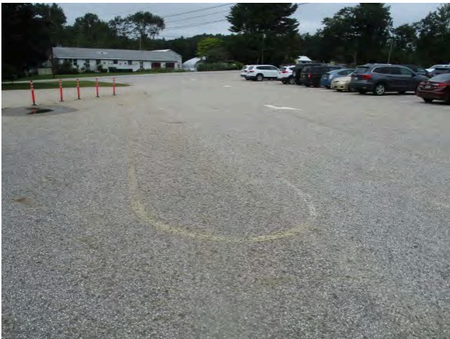
27. Pavement north of main entrance view north
