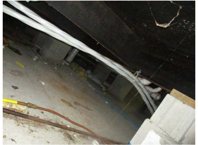
34. Crawlspace under 1996 addition
