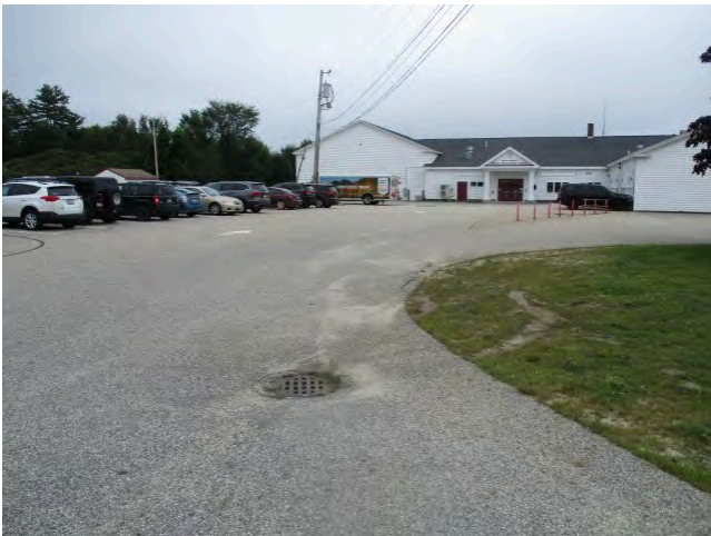
23. Pavement at east Property entrance from Shaw Hill Road
