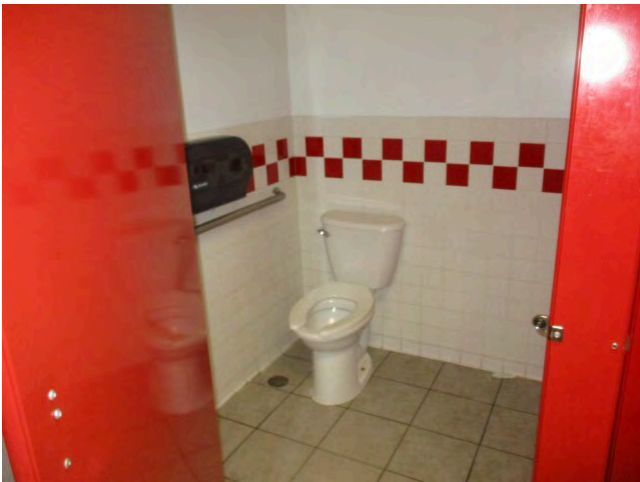
75. Boy's restroom near main office
