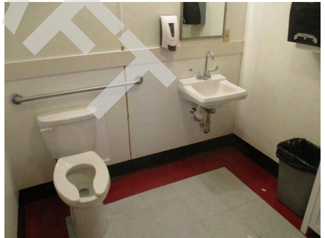
108. Restroom in 1996 addition
