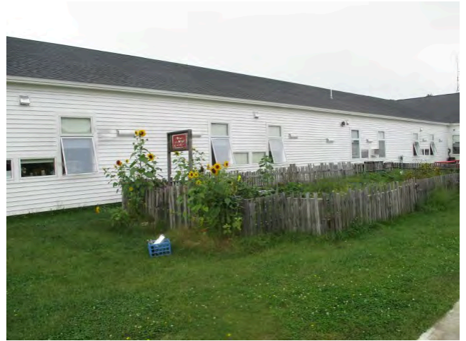
14. East elevation of south wing
