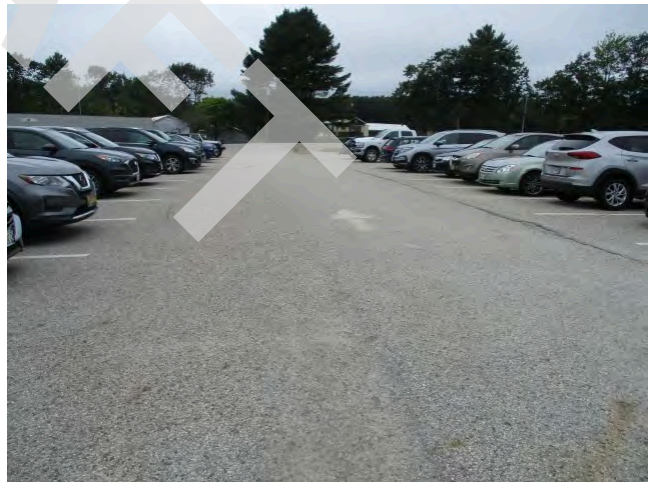
28. Pavement on east side of parking area view north
