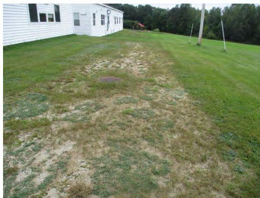
Septic tank on west side of building
