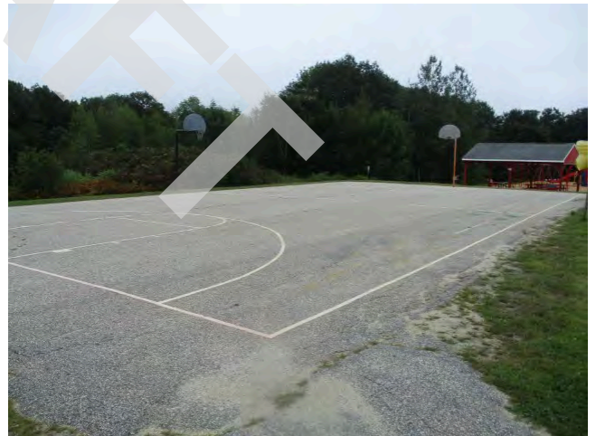
32. Basketball court west of 1996 addition
