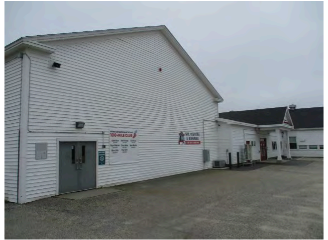
18. North elevation of gymnasium
