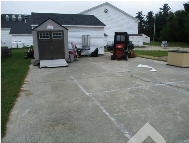
21. South elevation of maintenance building
