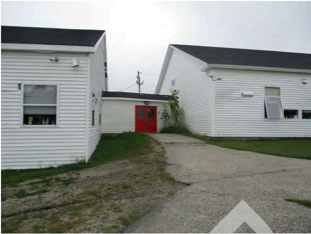
13. East elevation of connector to 1996 addition
