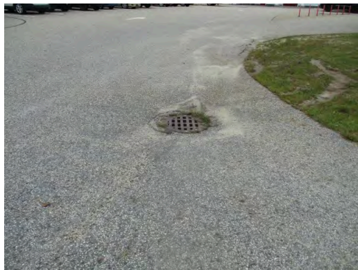
Catchbasin at east Property entrance
