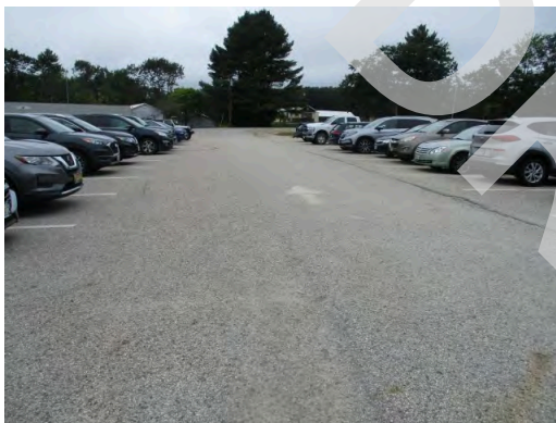
Pavement on east side of parking area view north
