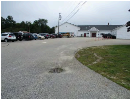
Pavement at east Property entrance from Shaw Hill Road
