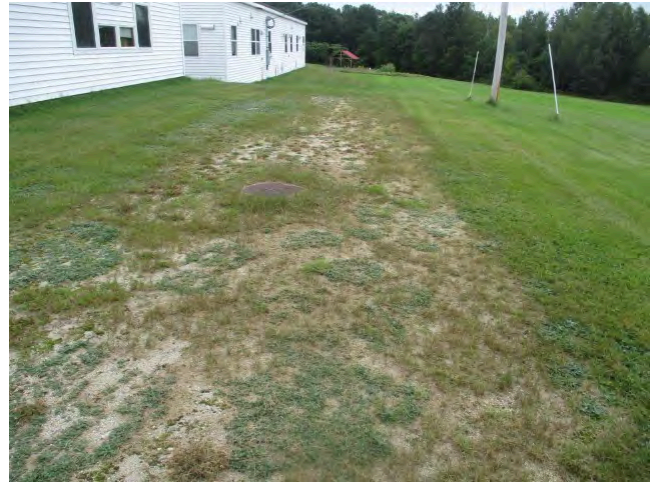
38. Septic tank on west side of building
