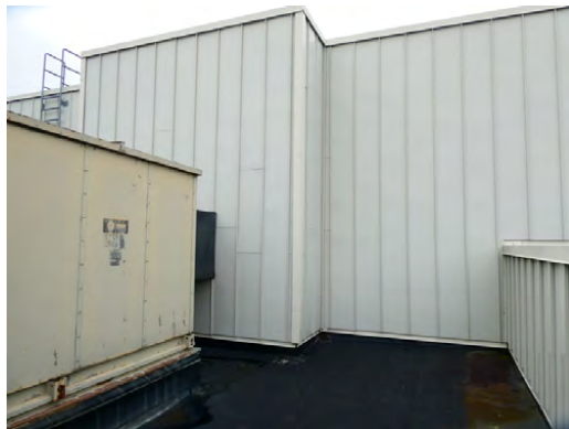
Exterior - Metal panels at south elevation (roofline)
