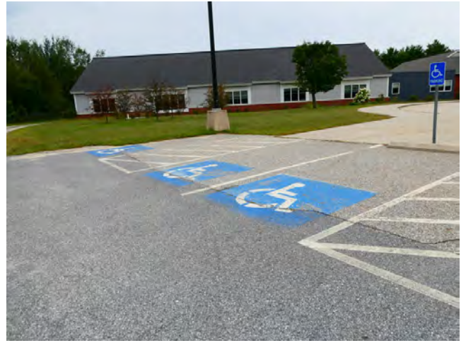
6. Site - Accessible parking spaces at main parking area
