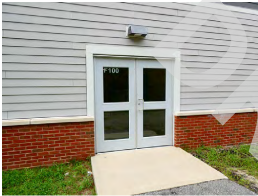
Exterior - Double secondary door type for middle school
