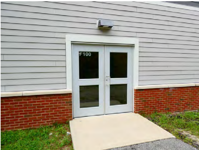
79. Exterior - Double secondary door type for middle school
