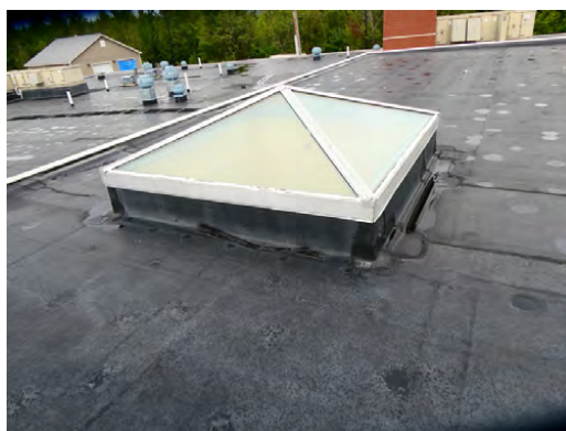
Roof - Curb mounted skylight type
