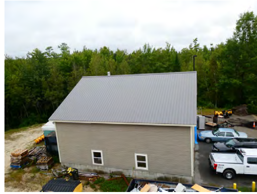
Roof - Metal roofing type for the biomass heating system building
