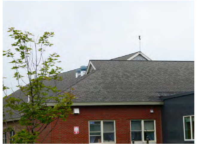
70. Roof - Pitched roofs for middle school with asphalt shingles
