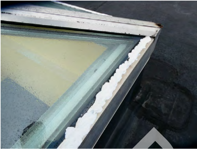
73. Roof - Skylights at central roof area with sealant replacement
