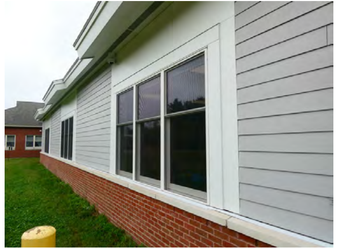
78. Exterior - Double hung window type for middle school
