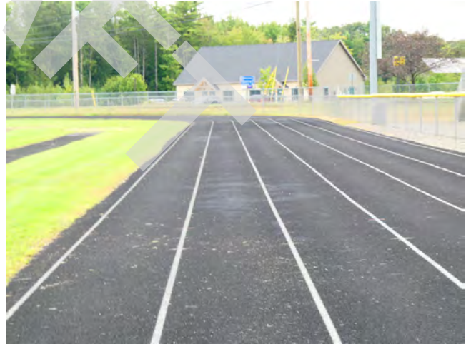
20. Site - Track surface condition
