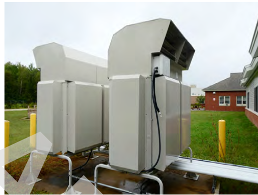
MEP - VRF heat pumps for the middle school
