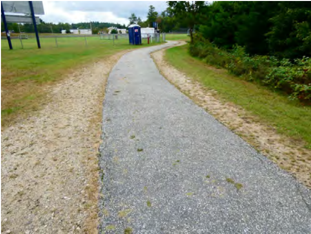
11. Site - Asphalt paved walkways to sports fields
