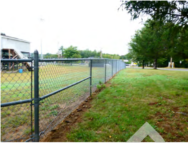
13. Site - Chain link perimeter fencing along track and football field
