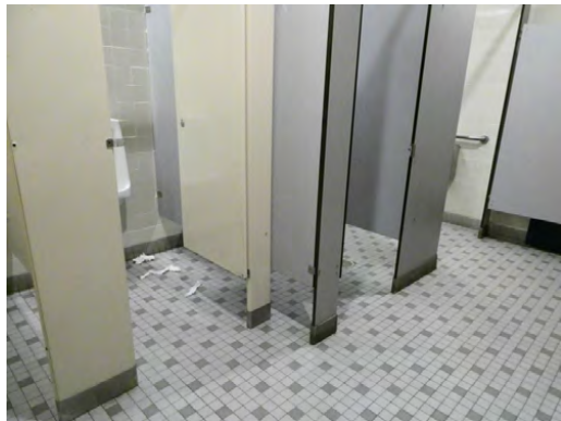
Interiors - Common area toilet room finishes and fixtures
