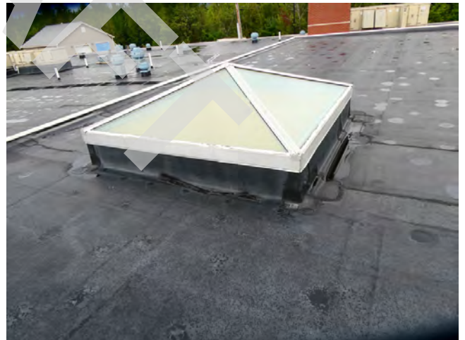
56. Roof - Curb mounted skylight type
