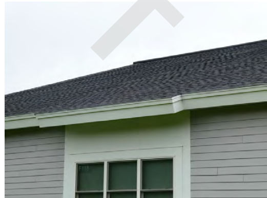
Roof - Pitched roofs for middle school with asphalt shingles
