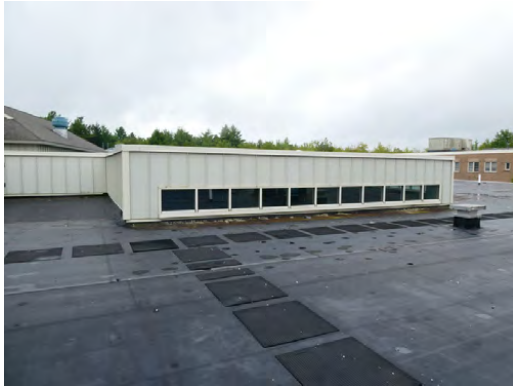
Exterior - Clerestory windows at roofline (west facing)
