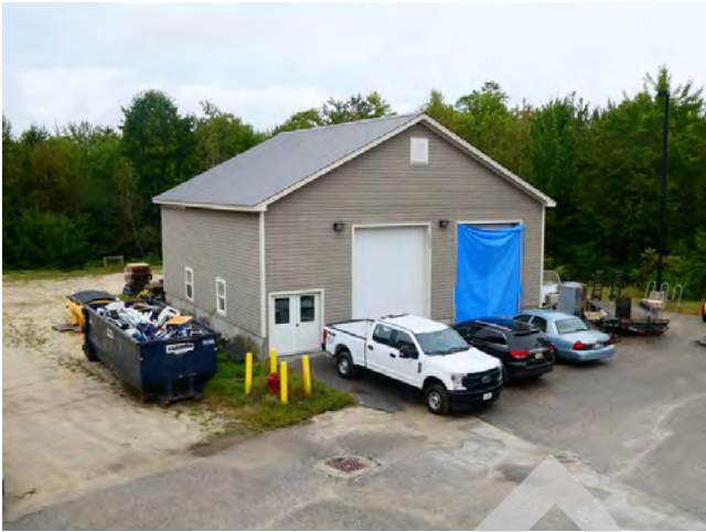
33. Exterior - Building for the biomass heating system
