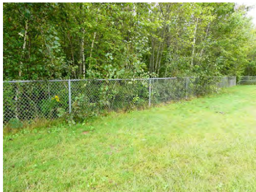
Site - Chain link fencing at south perimeter
