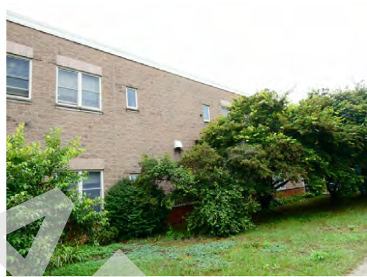
Exterior - Split face CMU facade finishes
