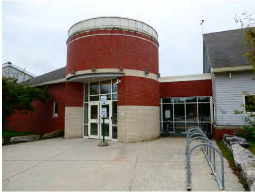
Exterior - Main entry to the middle school
