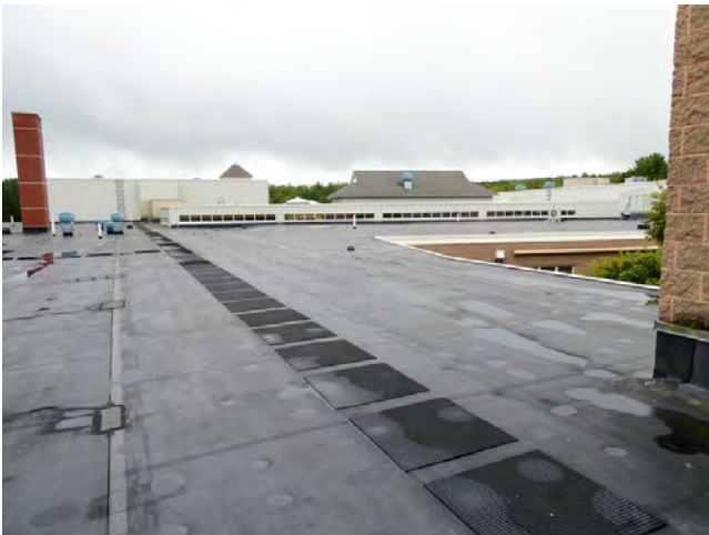
59. Roof - High school roof area facing east
