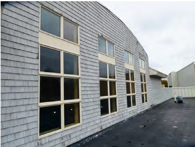
31. Exterior - Awning window type at roofline
