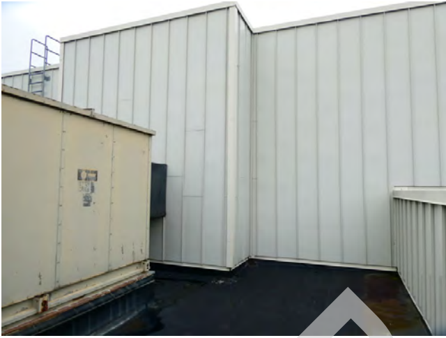
45. Exterior - Metal panels at south elevation (roofline)
