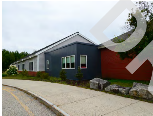
Exterior - Facade finishes for middle school
