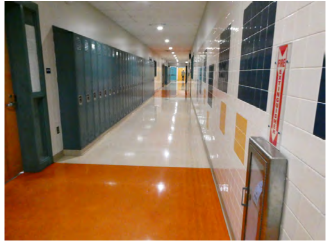
86. Interiors - Common area corridor finishes in high school
