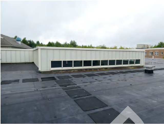
77. Exterior - Clerestory windows at roofline (west facing)
