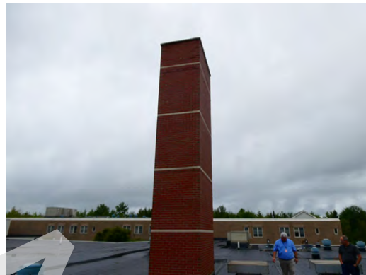
Roof - Brick clad chimney for the boilers
