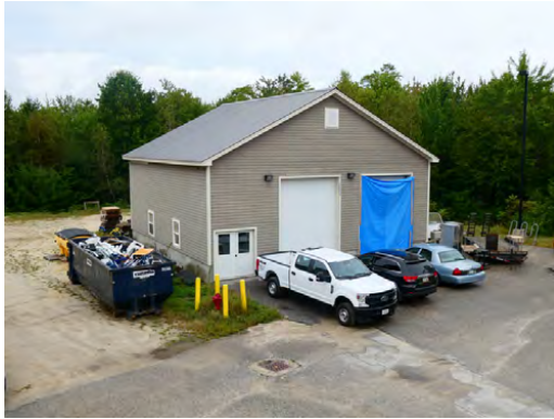
Exterior - Building for the biomass heating system
