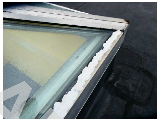
Roof - Skylights at central roof area with sealant replacement
