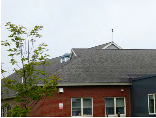
Roof - Pitched roofs for middle school with asphalt shingles
