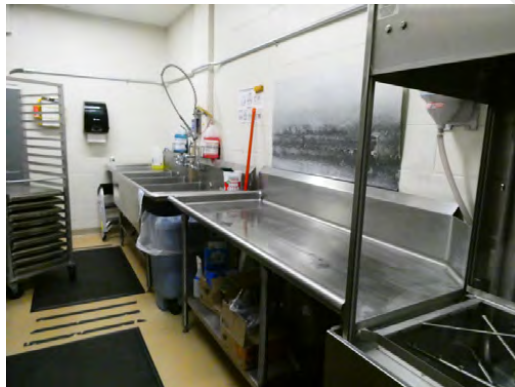
Interiors - Commercial kitchen finishes and equipment
