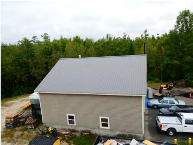
71. Roof - Metal roofing type for the biomass heating system building
