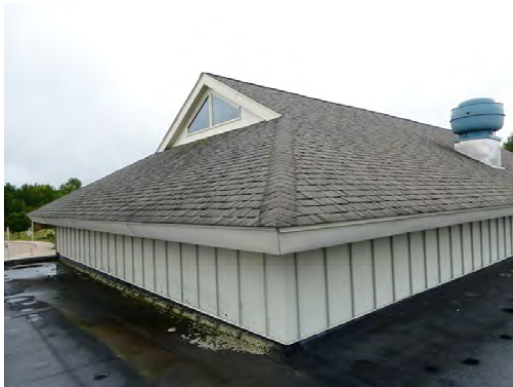
Roof - Pitched roof section with asphalt shingles (central roof)
