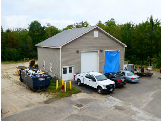
Exterior - Building for the biomass heating system
