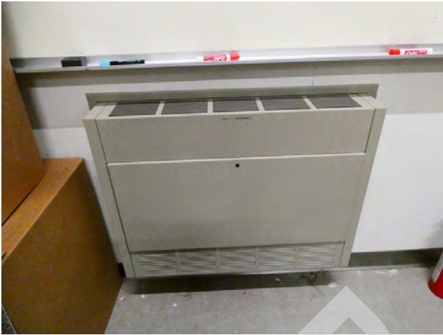
129. MEP - Wall mounted forced air cabinet unit
