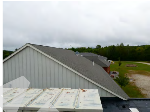
Roof - Overview of the middle school roof area
