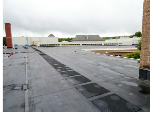
Roof - High school roof area facing east
