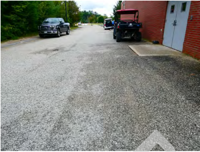
5. Site - Asphalt paved drives throughout
