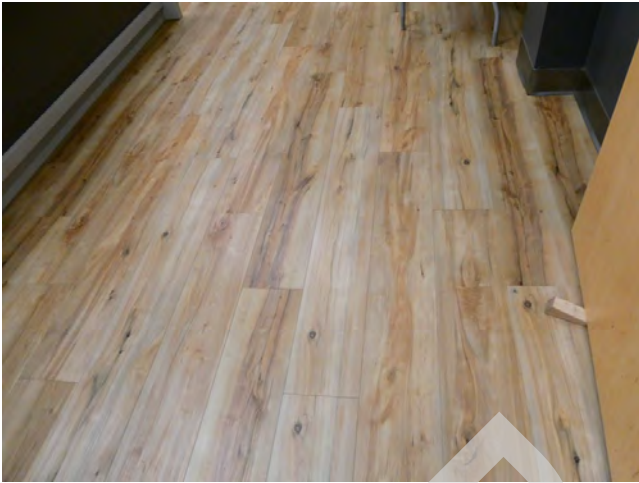
105. Interiors - Vinyl flooring type in middle school classroom
