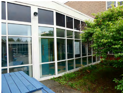
Exterior - Storefront glazing type at courtyard area
