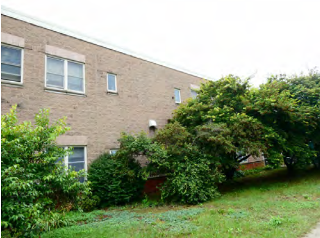
43. Exterior - Split face CMU facade finishes
