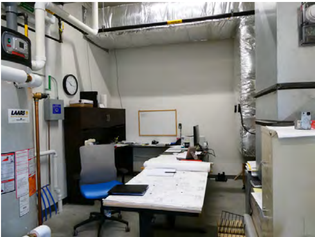
151. Interiors - Maintenance office finishes
