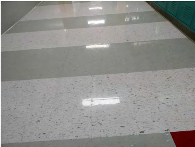
103. Interiors - VCT flooring in middle school common corridors
