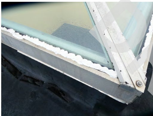
Roof - Skylights at central roof area with sealant replacement
