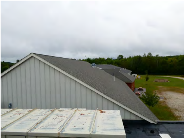
67. Roof - Overview of the middle school roof area
