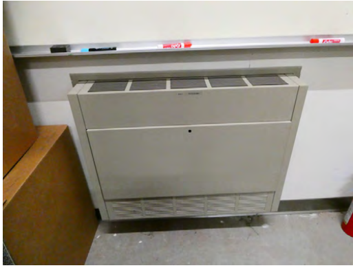
MEP - Wall mounted forced air cabinet unit
