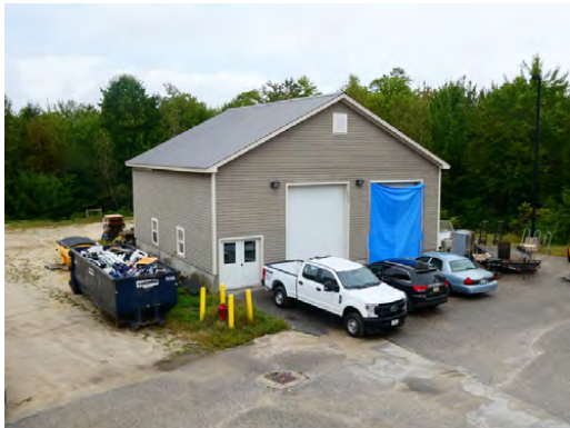
Exterior - Building for the biomass heating system
