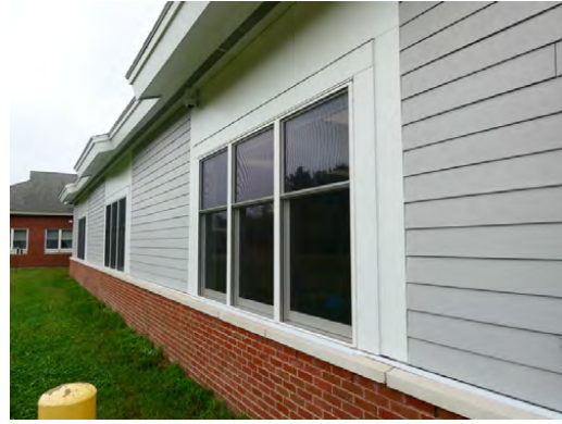
Exterior - Double hung window type for middle school
