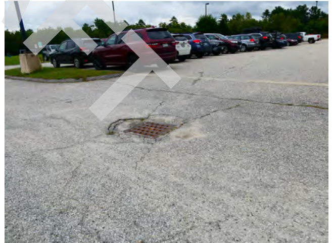
8. Site - Main parking surface condition
