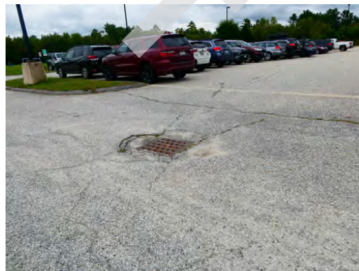
Site - Main parking surface condition
