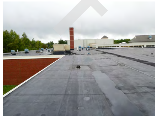
Roof - Mechanically fastened EPDM membrane
