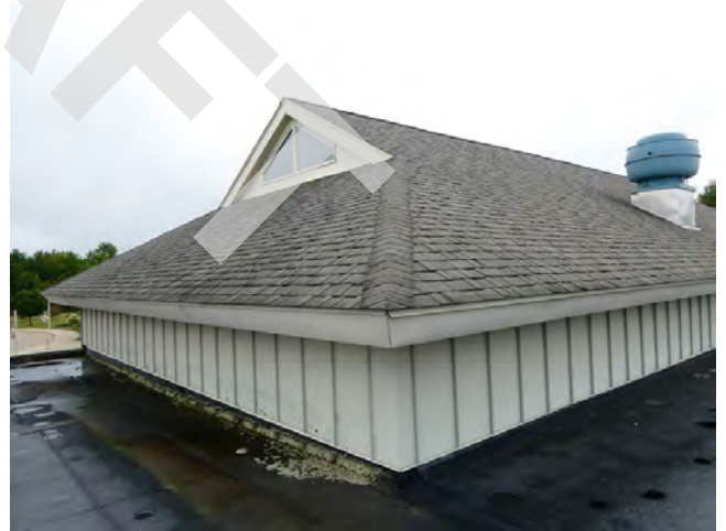
68. Roof - Pitched roof section with asphalt shingles (central roof)
