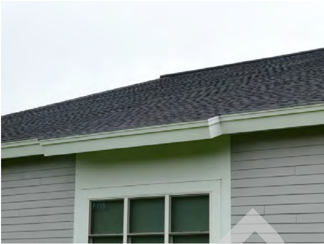
69. Roof - Pitched roofs for middle school with asphalt shingles
