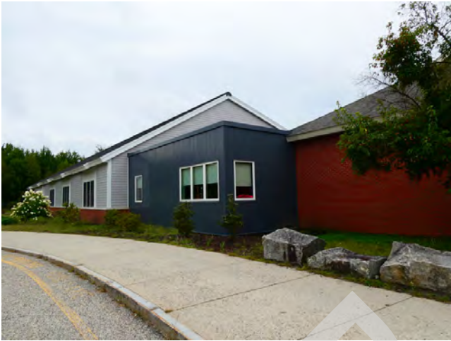
41. Exterior - Facade finishes for middle school
