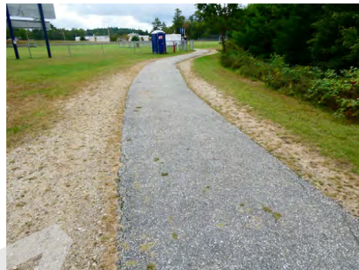
Site - Asphalt paved walkways to sports fields
