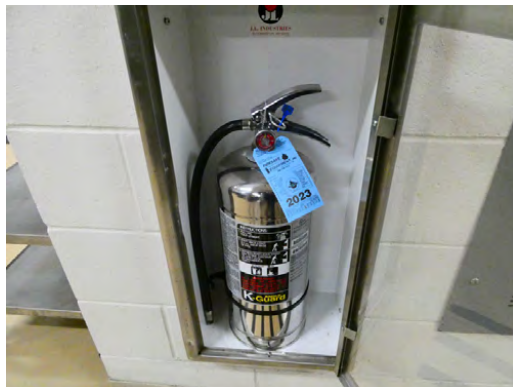
FLS - Chemical extinguisher in the commercial kitchen area
