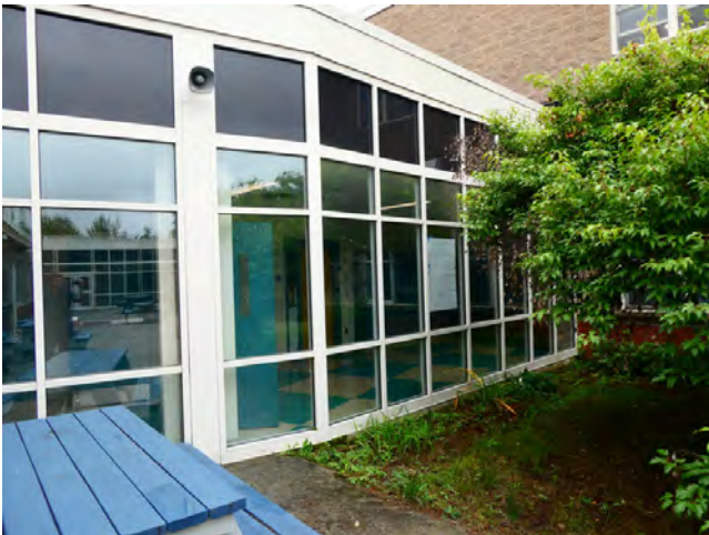
75. Exterior - Storefront glazing type at courtyard area
