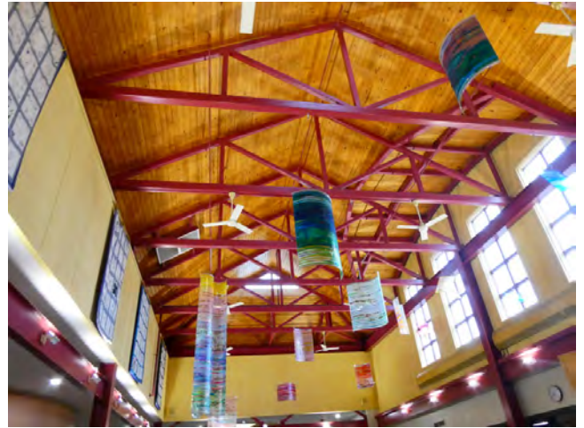
22. Structure - Steel framed joists in the central common area
