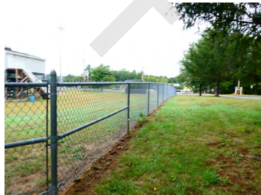
Site - Chain link perimeter fencing along track and football field
