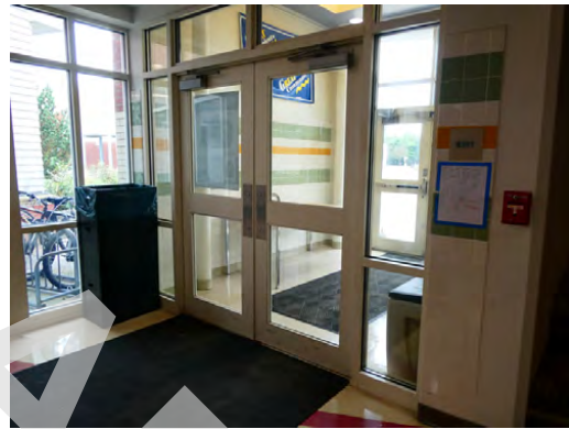
Interiors - Middle school entryway via storefront system
