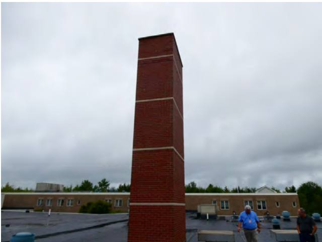
55. Roof - Brick clad chimney for the boilers
