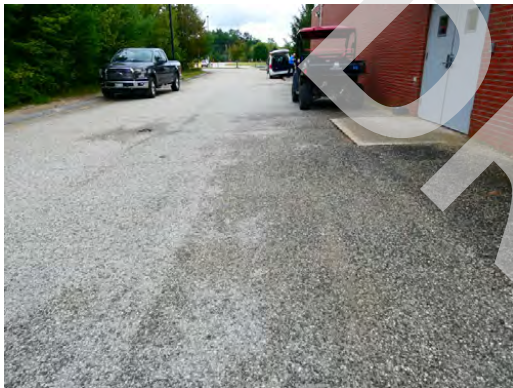
Site - Asphalt paved drives throughout
