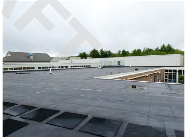
60. Roof - High school roof area facing south
