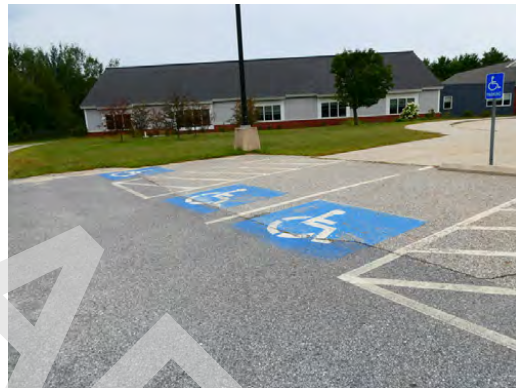
Site - Accessible parking spaces at main parking area
