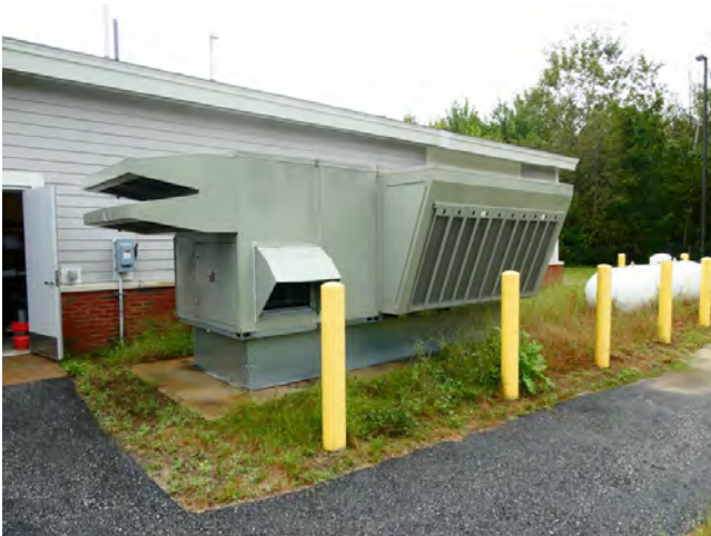
119. MEP - Packaged outdoor air unit for the middle school common areas
