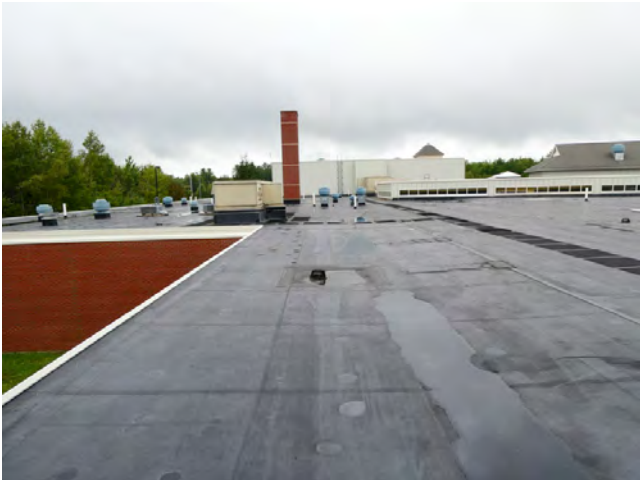
63. Roof - Mechanically fastened EPDM membrane
