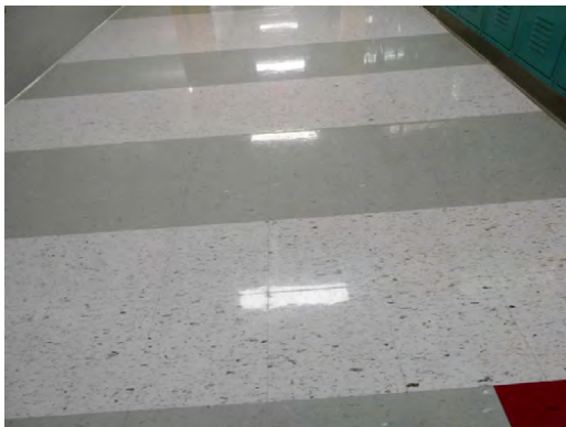
Interiors - VCT flooring in middle school common corridors
