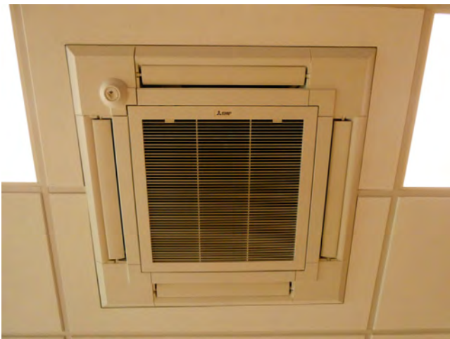
127. MEP - VRF interior unit type
