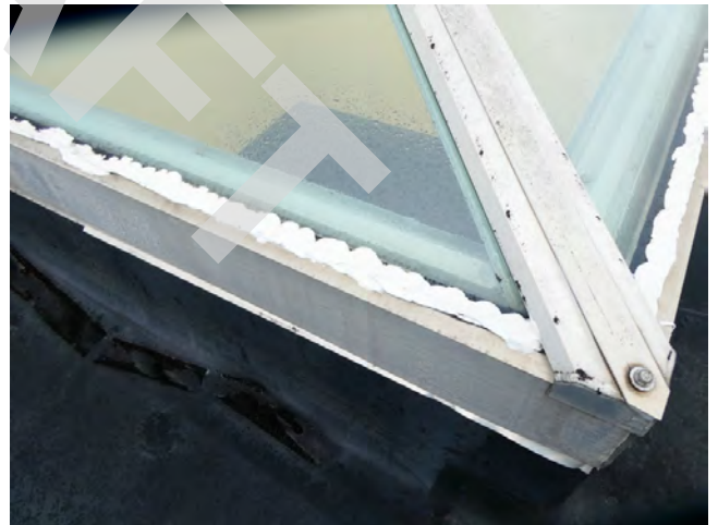
72. Roof - Skylights at central roof area with sealant replacement
