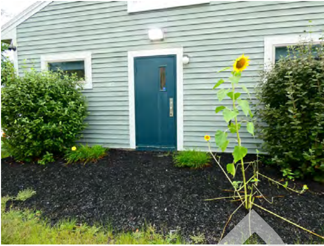
25. Exterior - Painted steel service door
