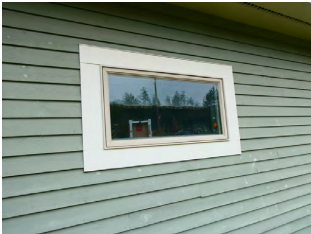
23. Exterior - Awning window type with vinyl framing
