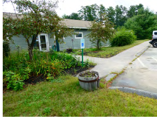
Site - Asphalt paved pedestrian walkway at south perimeter
