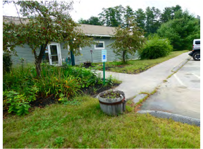
10. Site - Asphalt paved pedestrian walkway at south perimeter
