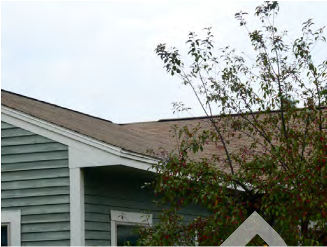
17. Roof - Pitched roof with composition asphalt shingles
