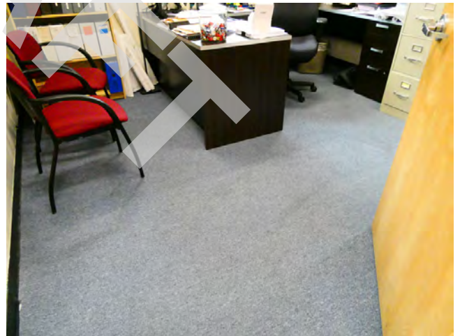
40. Interiors - Office with original carpeting type
