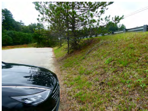
Site - Sloped grade along south perimeter
