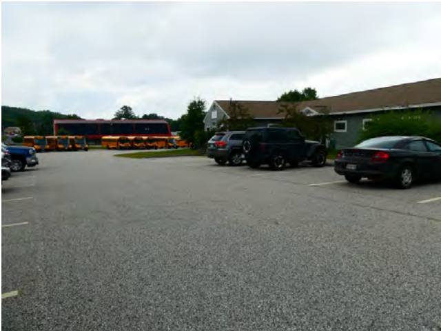
3. Site - South parking area and pavement condition
