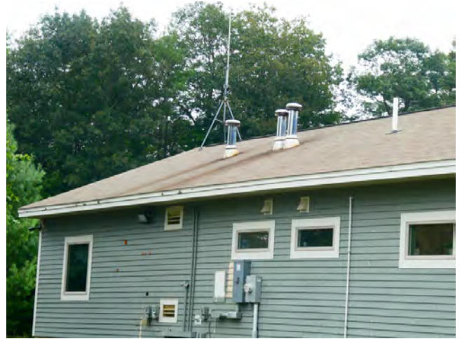
18. Roof - Pitched roof with composition asphalt shingles
