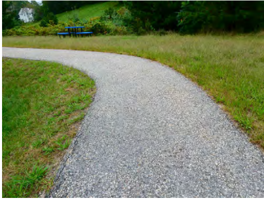
Site - Asphalt paved pedestrian walkway at north perimeter
