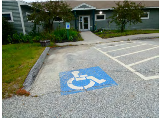
6. Site - Accessible parking space at main entrance
