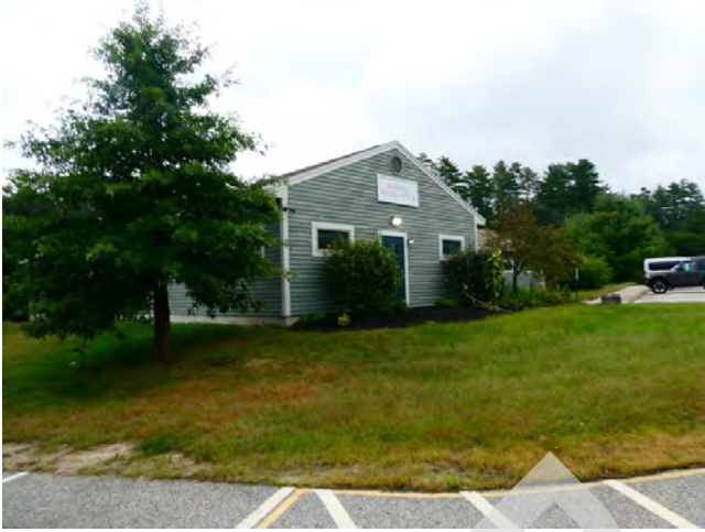
1. Overall view of the Subject Property
