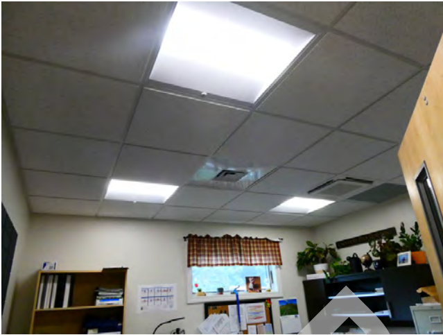
45. Interiors - Ceiling panel finish type
