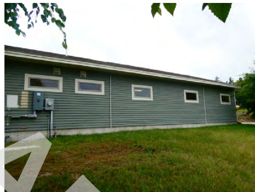
Elevations - West facing elevation
