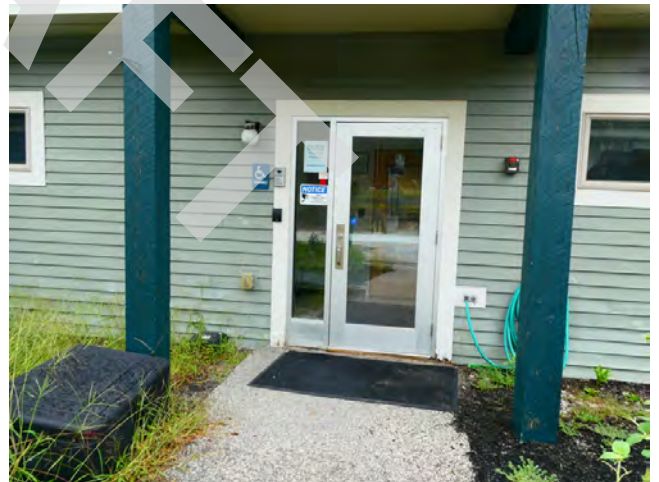
24. Exterior - Main entrance along south elevation
