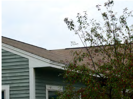
Roof - Pitched roof with composition asphalt shingles
