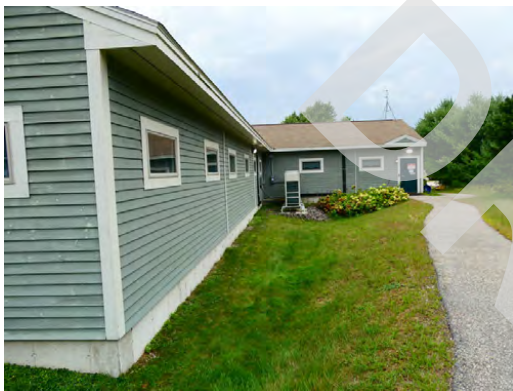
Elevations - North facing elevation
