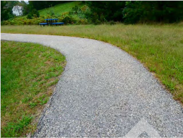
9. Site - Asphalt paved pedestrian walkway at north perimeter
