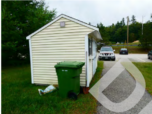
Site - Storage structure along the east perimeter
