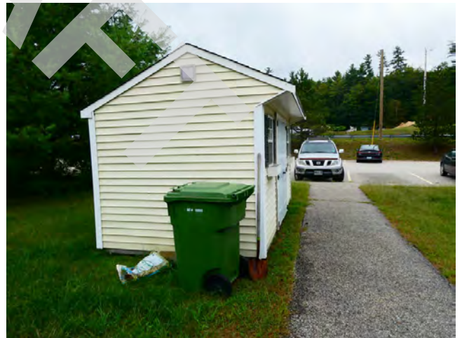
12. Site - Storage structure along the east perimeter
