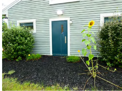
Exterior - Painted steel service door
