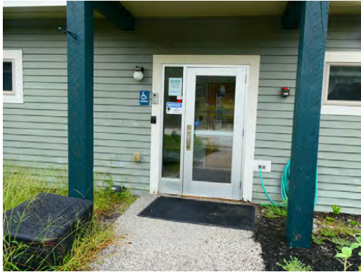
Exterior - Main entrance along south elevation
